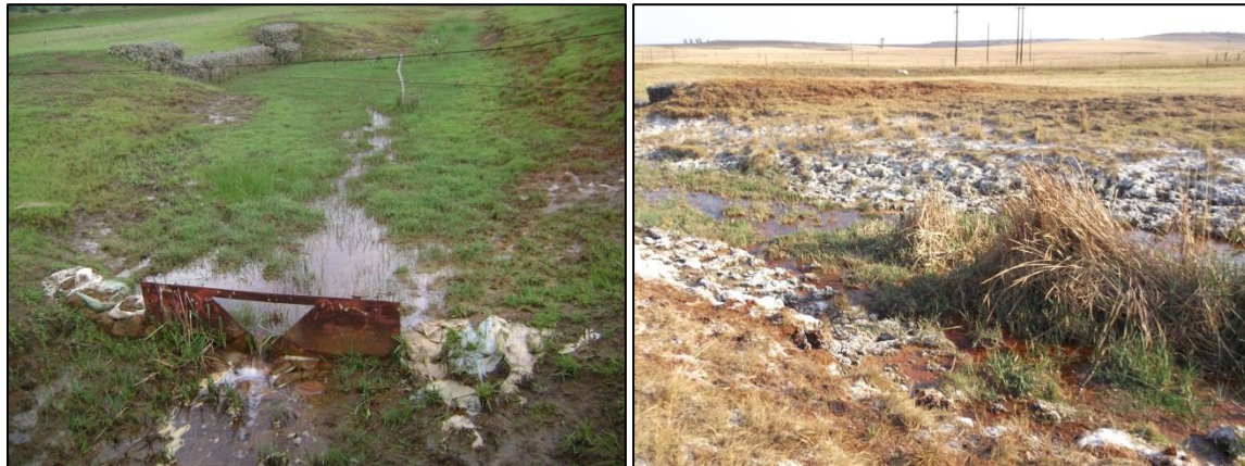
Figure 5-8: Decant emanating southeast of the Discard Dump
