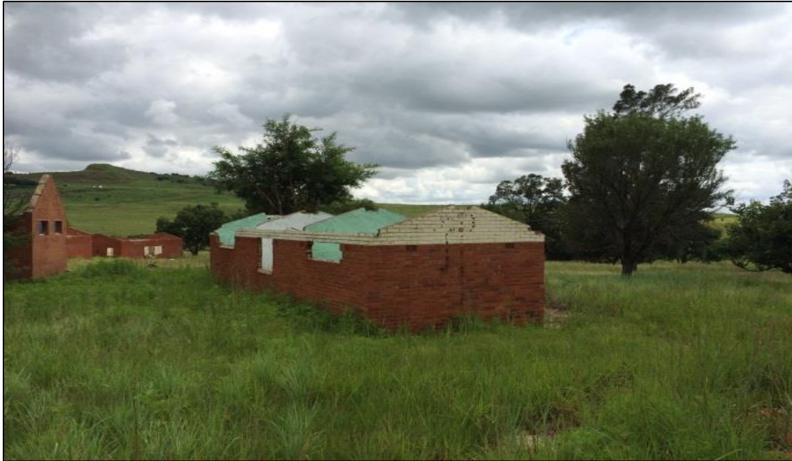
Figure 5-5: Remnant infrastructure north of the Discard Dump
