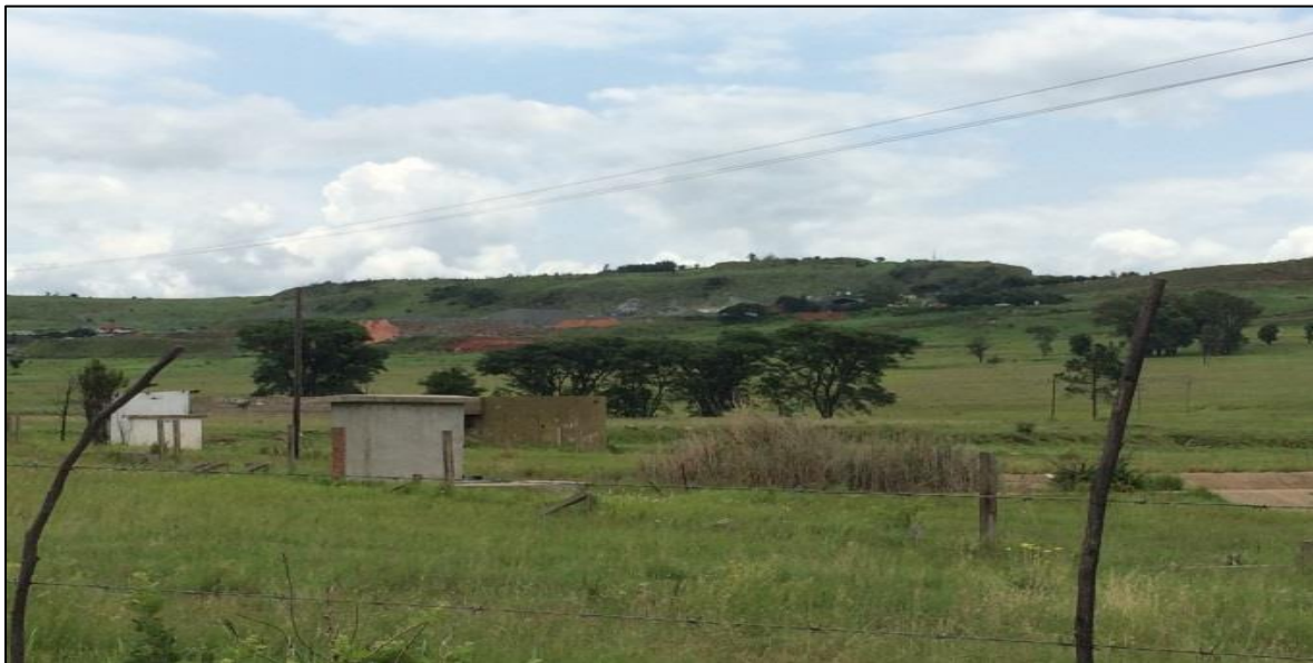
Figure 5-6: Decommissioned WWTP north of the Discard Dump
