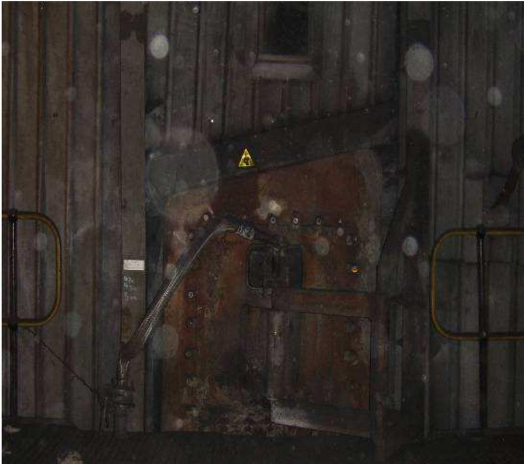
**Figure 1 Boiler (lower portion) with the brine injection nozzle**
