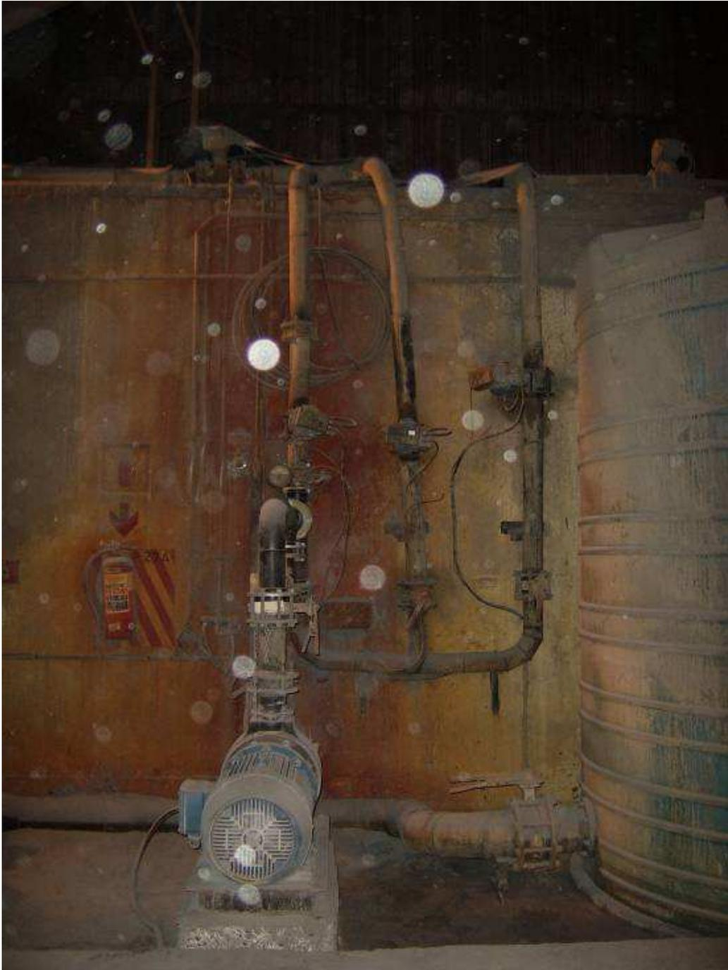
**Figure 3 Brine injection tank (left) with pump (centre) at boiler 2**
