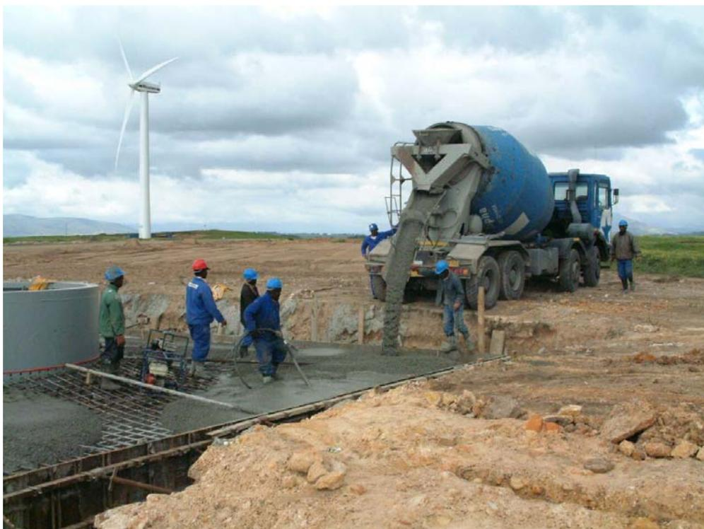
**Figure 7.1:** Photograph illustrating the construction of the foundation of one of the turbines at the Klipheuwel demonstration facility (photo courtesy of Eskom)
