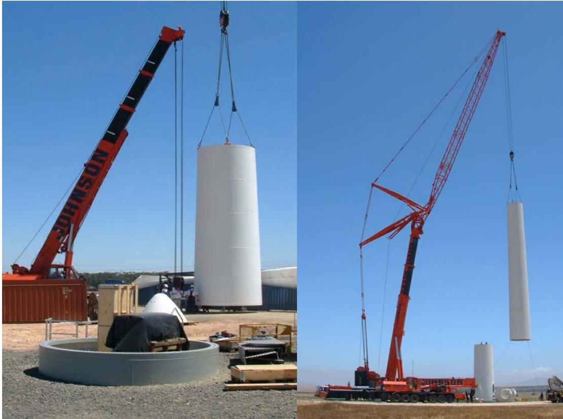
**Figure 7.3:** Photograph illustrating the assembly of a turbine tower utilising a large lifting crane (photographs courtesy of Eskom taken during the construction of the Klipheuwel demonstration facility)
