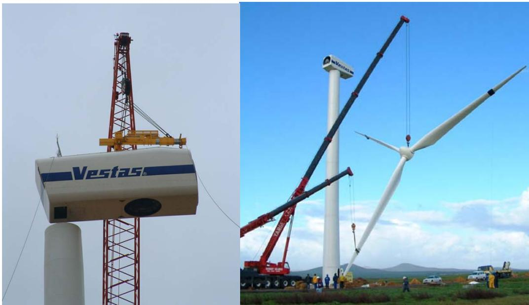
**Figure 7.4:** Photograph illustrating the assembly of a turbine (nacelle and blades) utilising a large lifting crane (photographs courtesy of Eskom from construction at the Klipheuwel demonstration facility)
