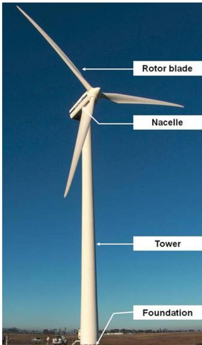
**Figure 3.4:** Illustration of the main components of a wind turbine
