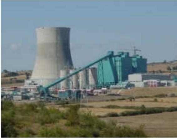
**Figure 4.7** Photograph showing a power station with the dry cooling tower of the Stack-in-Tower system of indirect dry cooling technology
