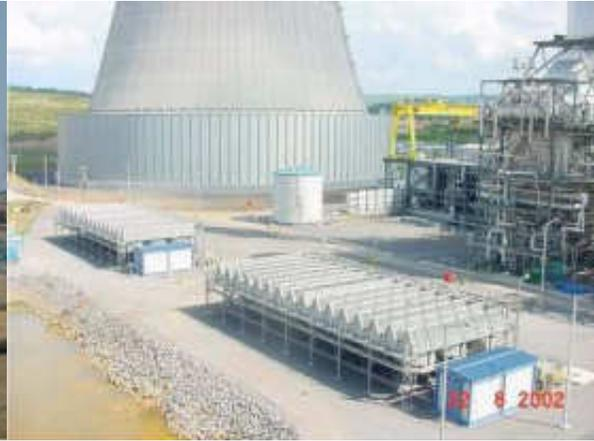
**Figure 4.8** Photograph showing a power station with the water-to-air heat exchangers of the Stack-in-Tower system of indirect dry cooling technology
