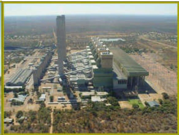
**Figure 4.5 Photograph showing a power station with indirect dry cooling technology**
