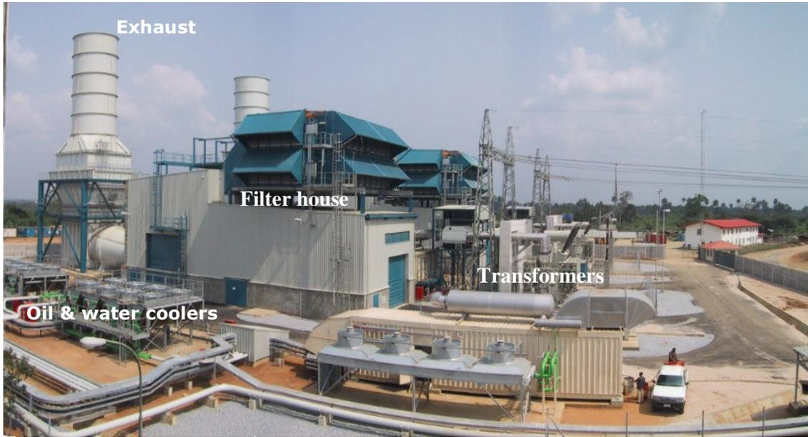
**FIGURE 3** Example of two OCGT power generation units
