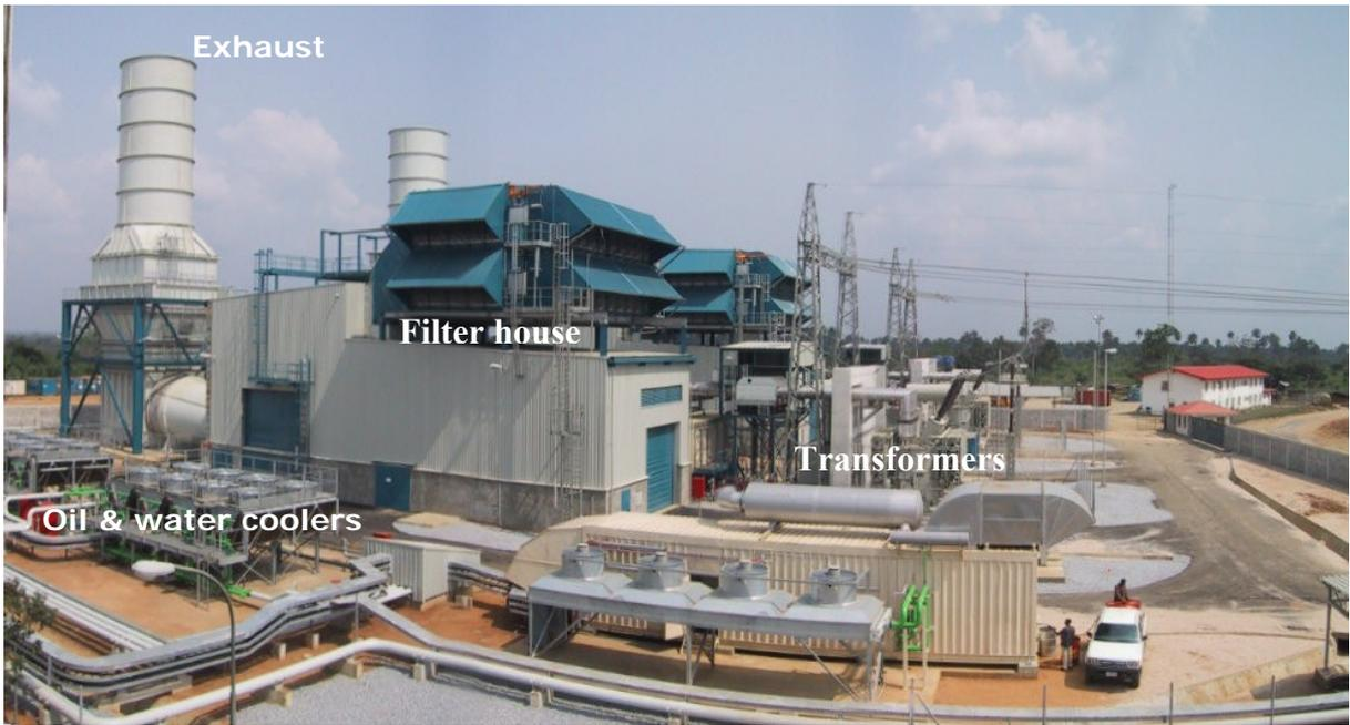
**FIGURE 2** Example of two OCGT power generation units
