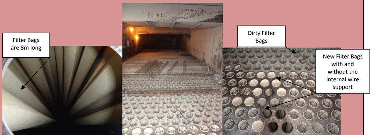
**Figure 5:** Inside a typical fabric filter plant
