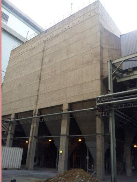
**Figure 2:** Existing Concrete ESP Casing within which the new Fabric Filter Plant will be installed, while extending the height of the casing with 1.1 meters.
