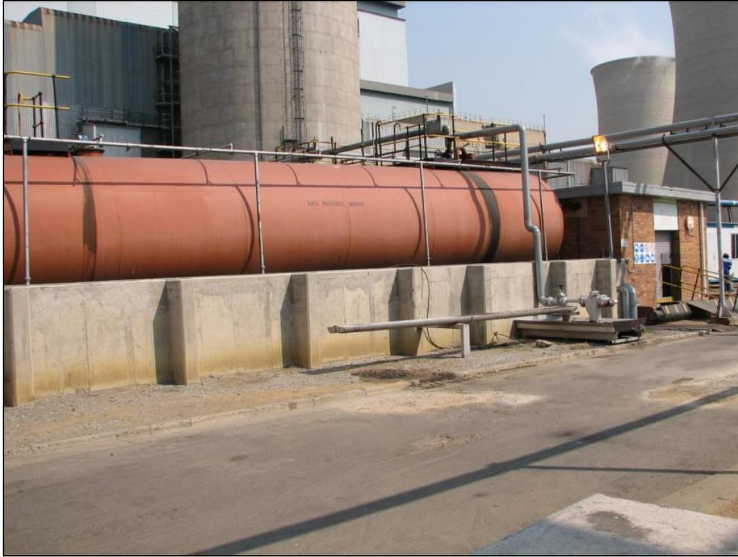
**Figure 3: Photo of an existing fuel storage tank at the Grootvlei power station.**
