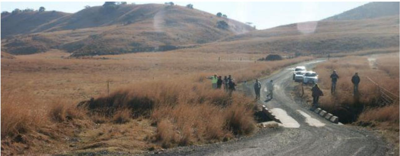
The existing road is a gravel road of approximately 7 – 8 metres in width. For a gravel road it is in fair to good condition, although with some signs of wear from traffic. The existing crossing of the Braamhoekspruit is a 5 metre wide (single lane) low level bridge, which is placed at right angles to the stream flow, resulting in rather poor horizontal alignment of the approaches to the crossing.
