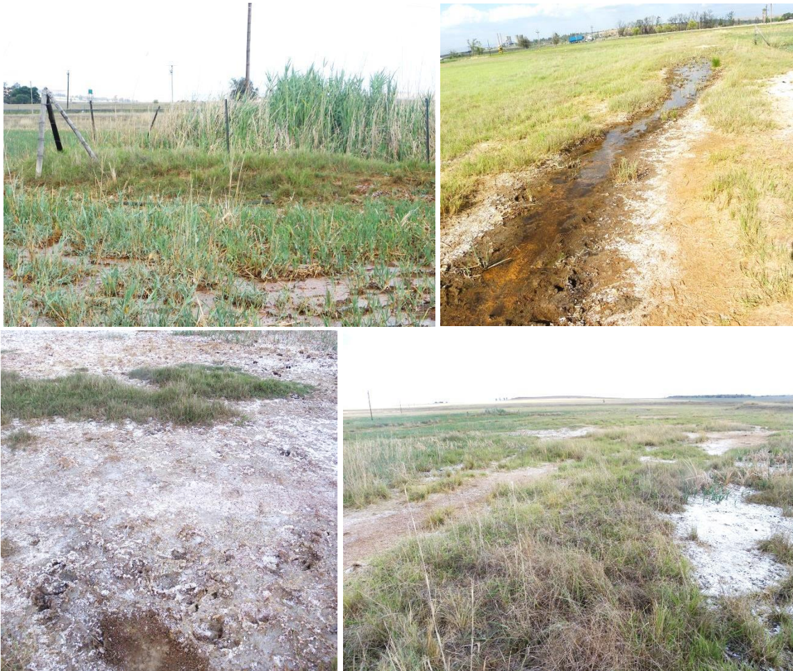
Figure 3-2: The decant locations and effects on site
