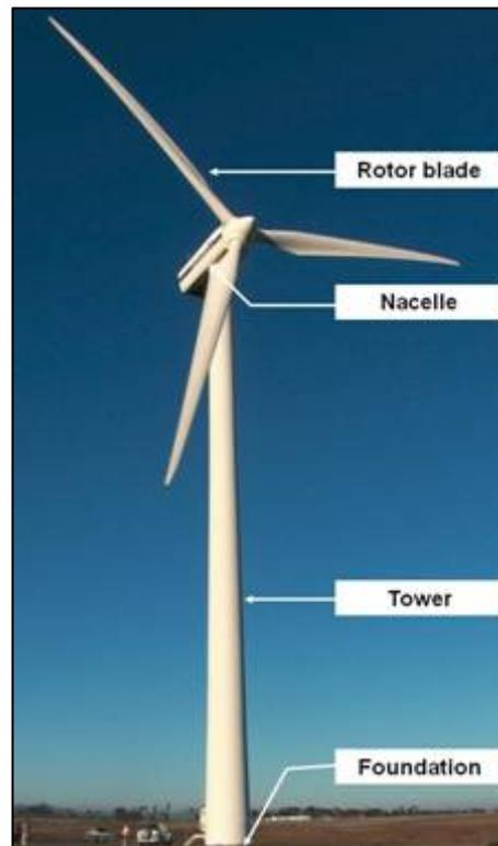
**Figure 1:** Illustration of the main components of a wind turbine<sup>1</sup>
