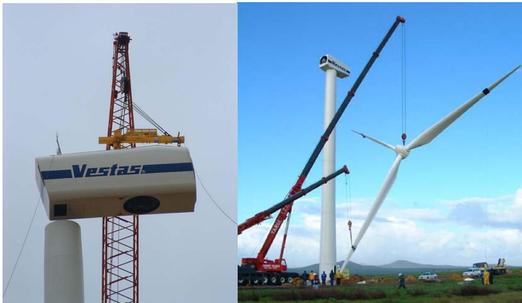
**Figure 7.6:** Photograph illustrating the assembly of a turbine (nacelle and blades) utilising a large lifting crane (photographs courtesy of Eskom from construction at the Klipheuwel demonstration facility)
