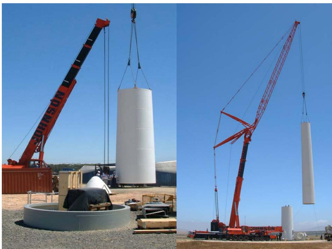
**Figure 7.5:** Photograph illustrating the assembly of a turbine tower utilising a large lifting crane (photographs courtesy of Eskom taken during the construction of the Klipheuwel demonstration facility)
