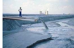
Ash dam showing ash mixed with water being pumped into the pond on top of the dam. The ash originates from the coal-burning power station nearby. The ash settles out and the water is recycled.
