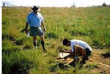
A rehabilitated ash dam. Once the ash dam reaches a certain height level in height, then rehabilitation will be carried out by putting on a layer of top soil and sowing various grasses. In the foreground is the grassy plateau of a vegetated ash dam. In the background is the Hendrina Power Station.
