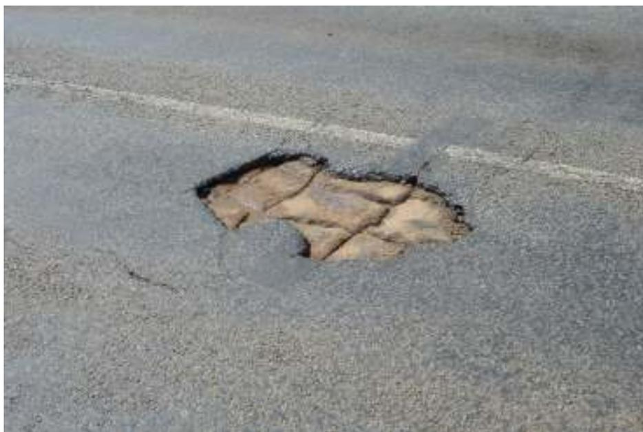
**Figure 4.2: Pothole on the R545 road**
