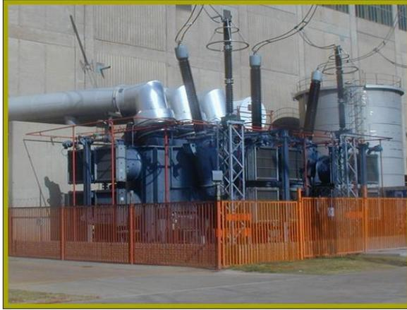
**Photo 10:** Step up transformers. The silver pipes enclose the conduits transporting electricity from the generator to the transformers (painted blue in the photograph)
