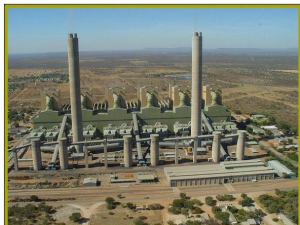
**Photos 3 and 4:** A typical direct dry cooled power station, without cooling towers
