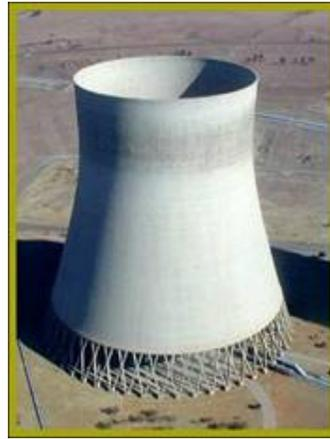
**Photos 5:** A typical indirect dry cooled power station, with cooling towers
