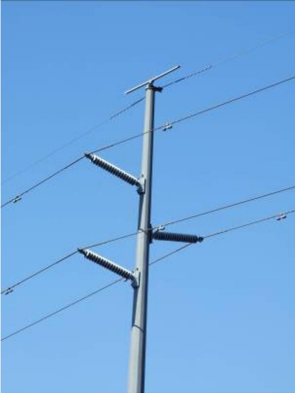
Figure 4: Single steel pole 88/132kV sub-transmission structure
