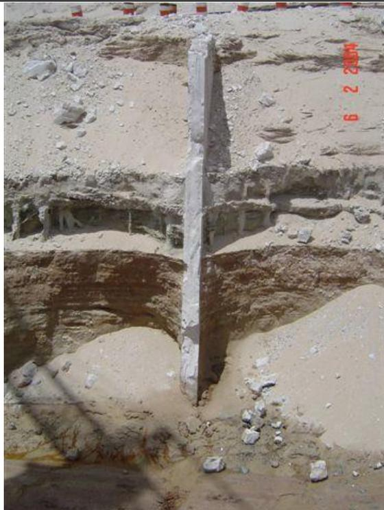
**Section of the Slurry Cut-Off Wall Exposed in the Excavation**
