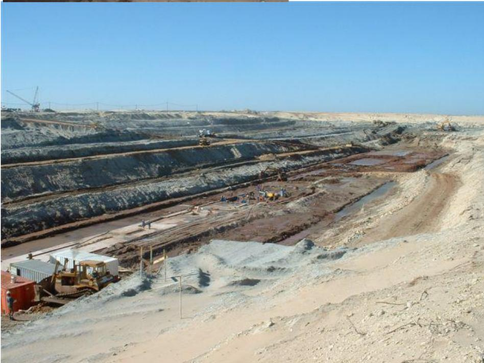
**View of the Main Harbour Excavation Showing Central Foundations and Stepped Benches**
