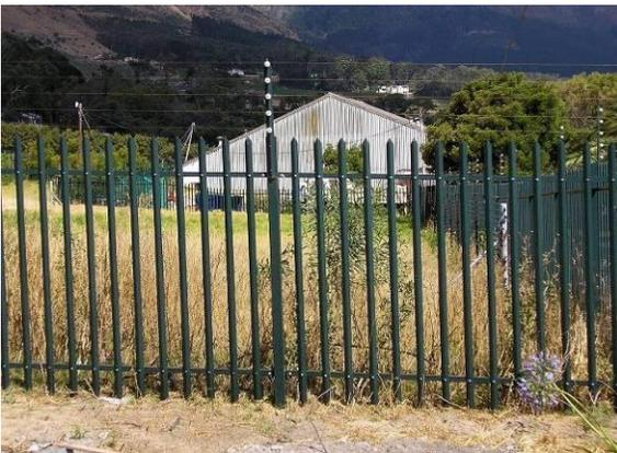
The palisade fence is OK, but the electrified wires at the top are not visible enough and therefore pose a threat to birds.
