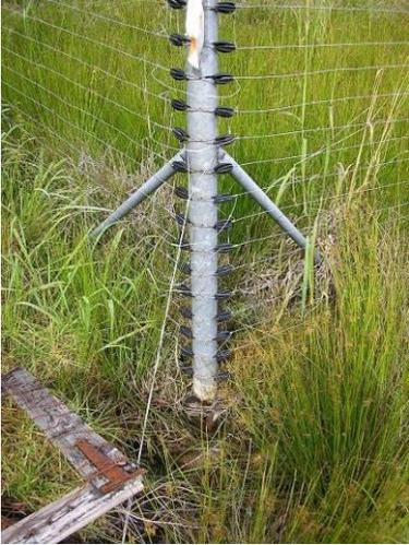
This type of electrified fence is an unmitigated disaster! Note the small gaps between strands and the many electrified strands near ground level.
