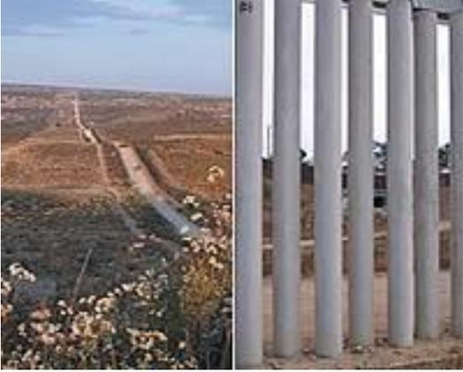
Photos of US-Mexico border fences taken in July 2006. (a) Border fence located east of San Diego, CA. (b) Recently built "permeable" border barrier located south of San Diego will allow migration of smaller species, but proposed double-barrier impermeable fencing may not.
