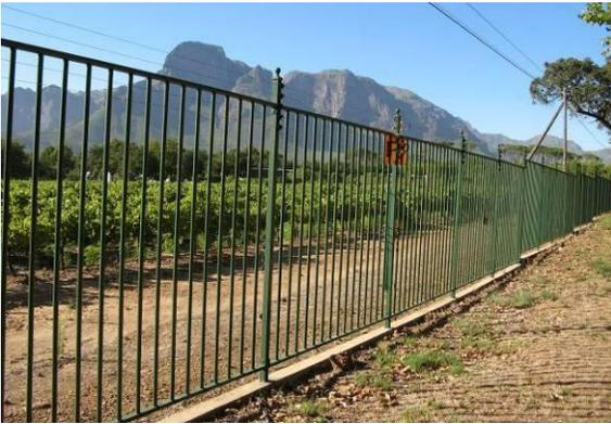
This palisade fence would be good if the concrete wall at the bottom were flush with the ground.
