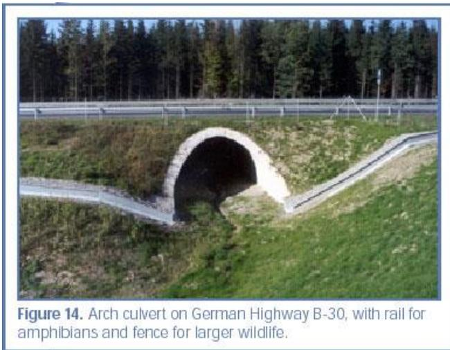
**Figure 14.** Arch culvert on German Highway B-30, with rail for amphibians and fence for larger wildlife.
