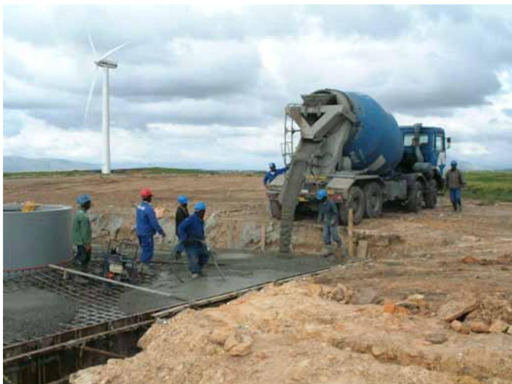
**Figure 5.5:** Photograph illustrating the construction of the foundation of one of the turbines at the Klipheuwel demonstration facility (photo courtesy of Eskom)
