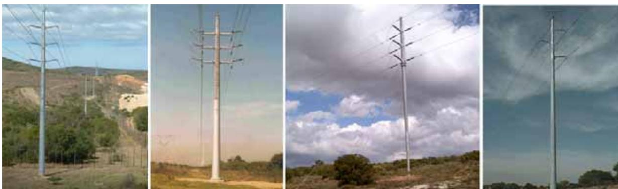
**Figure 5.10:** Examples of the proposed 132 kV monopole double circuit power line tower type.
