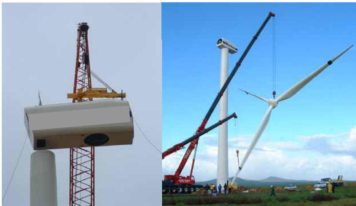
**Figure 5.8:** Photograph illustrating the assembly of a turbine (nacelle and blades) utilising a large lifting crane (photographs courtesy of Eskom from construction at the Klipheuwel demonstration facility)
