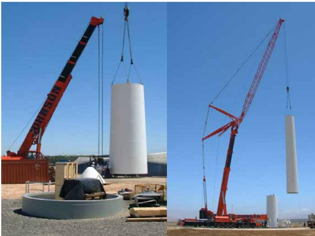
**Figure 5.7:** Photograph illustrating the assembly of a turbine tower utilising a large lifting crane (photographs courtesy of Eskom taken during the construction of the Klipheuwel demonstration facility)
