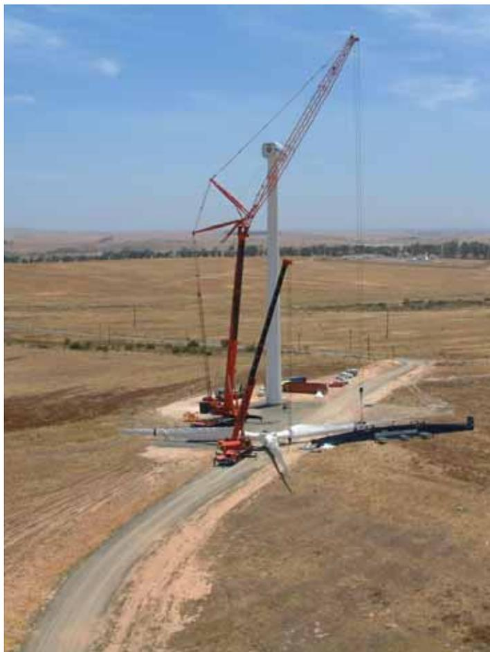
**Figure 5.4:** Photograph illustrating the laydown areas required during the erection of one of the turbines at the Klipheuwel demonstration facility (photo courtesy of Eskom)
