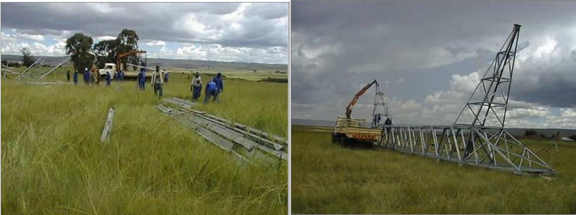
*Figure 27: Delivery of steel (left) and assembly of tower (right)*
