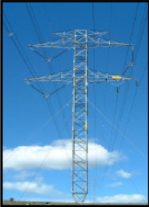
Photo 2: Self - supporting double circuit suspension tower.
