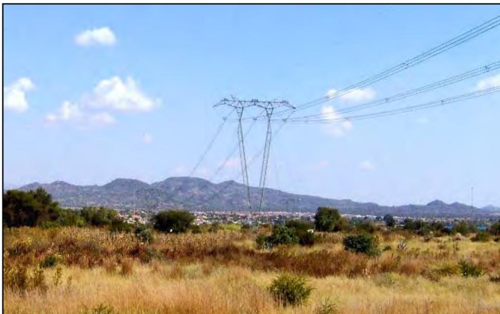
**Figure 2.7:** Guyed and Compact Cross-roped suspension tower typically used along the existing Dinaledi-Anderson 400kV transmission power line route
