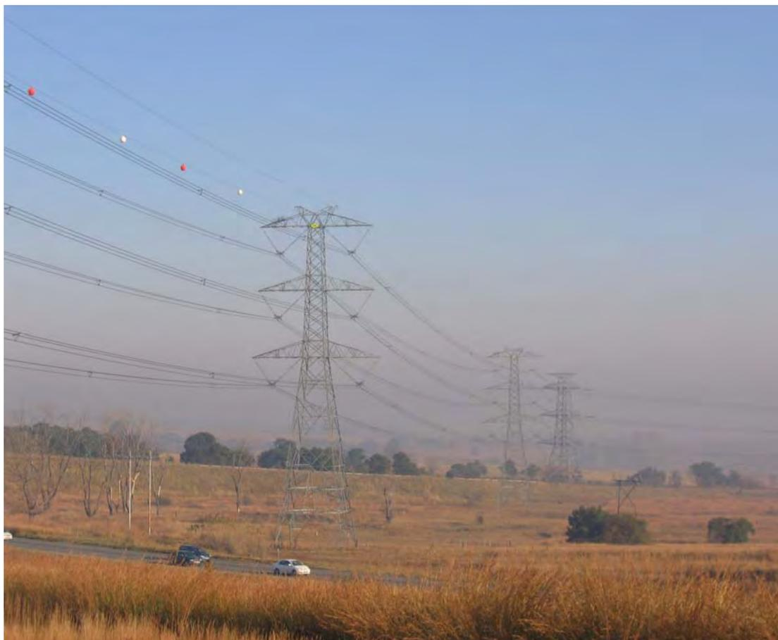
**Figure 2.6:** Self-supporting double-circuit tower
