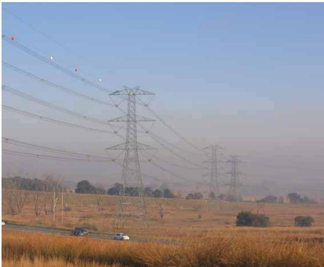
**Figure 2.6:** Self-supporting double-circuit tower
