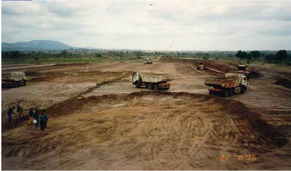
**Photograph 2.1:** showing earthworks for a substation site
