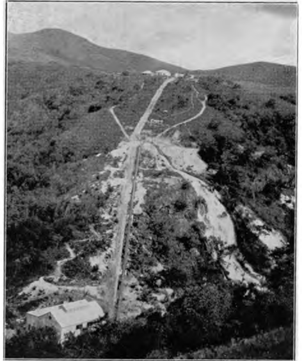
Sabie Gorge Scheme—Pipe Line and Power Station.
