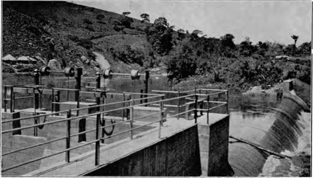
Sabie Gorge Scheme—Diversion Weir and Intake Works.
