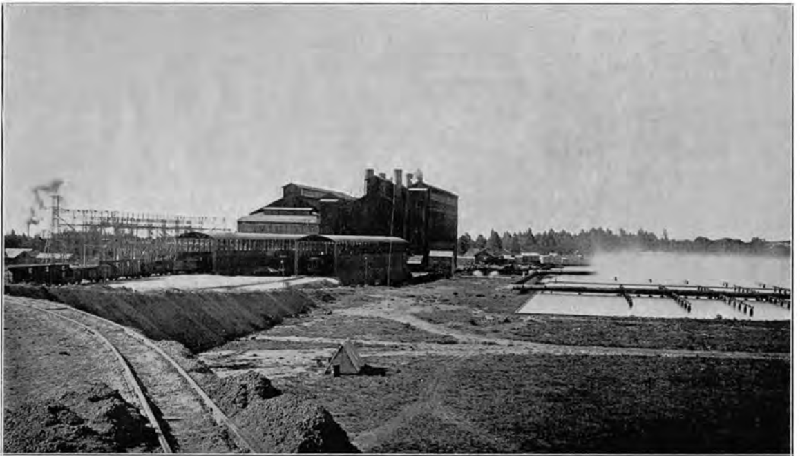
Witbank Power Station—Coal Staithees and Spray Ponds in Foreground.
