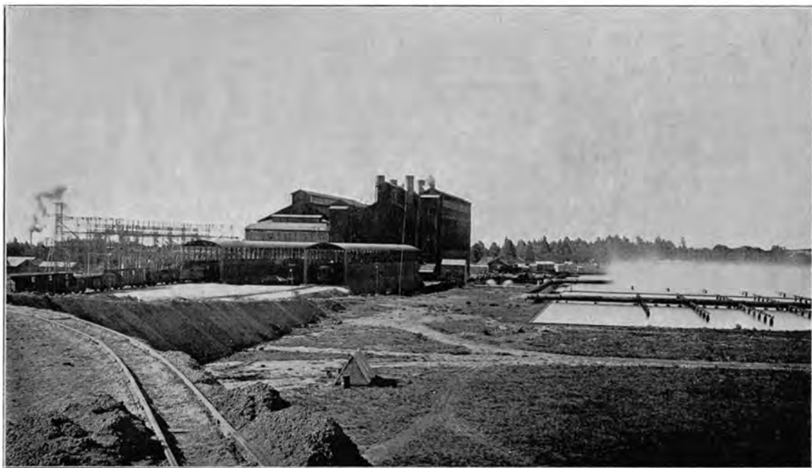
Witbank Power Station—Coal Staithe and Spray Ponds in Foreground.
