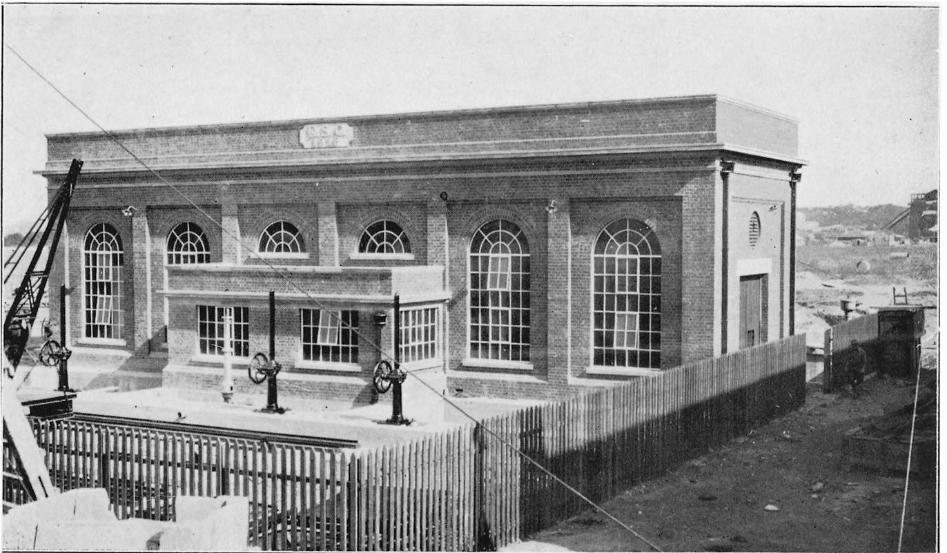
Durban Undertaking—Pump House.
