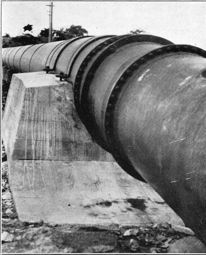
Sabie Undertaking—42in. Pressure Pipe.
