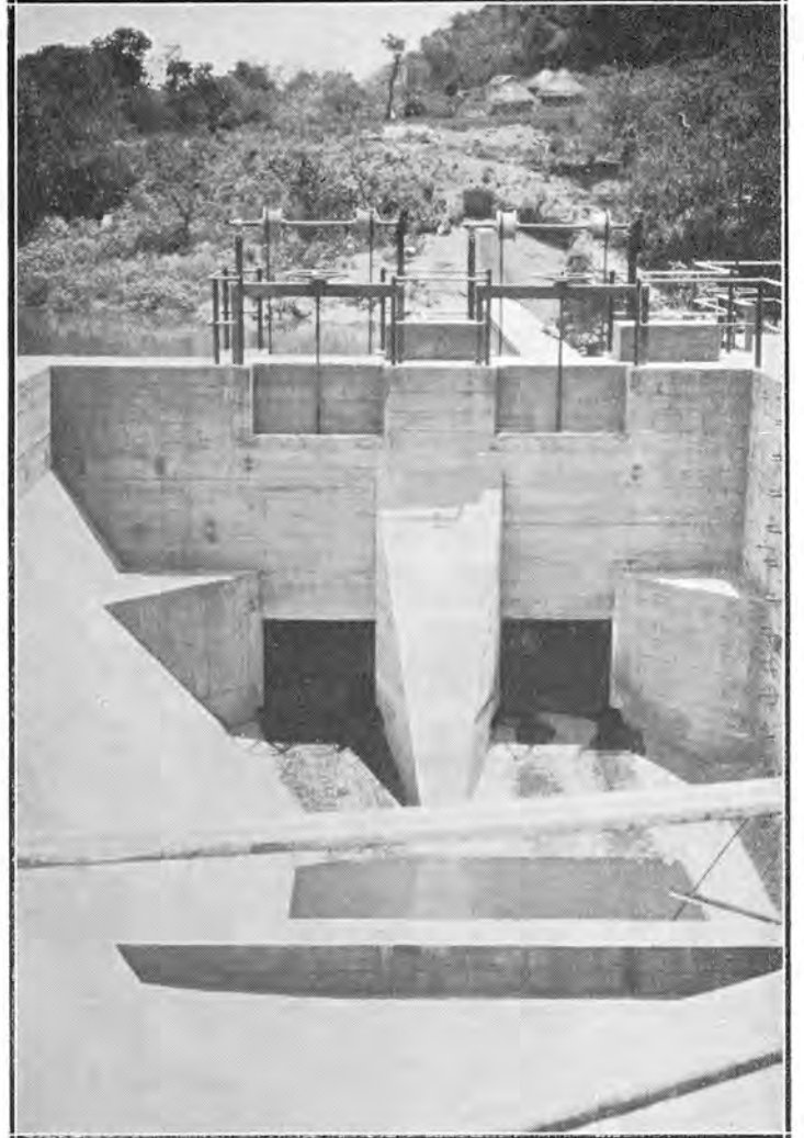
Sabie Undertaking—Settling Basin at Intake Works.
