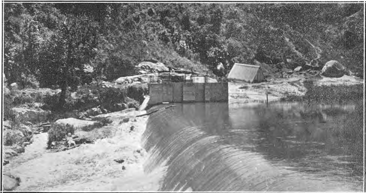
Sabie Undertaking—Diversion Weir.
