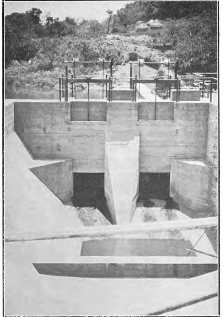
Sabie Undertaking—Settling Basin at Intake Works.
