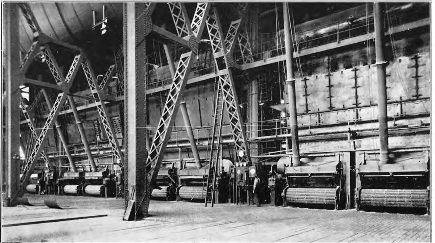
Capetown Undertaking: Salt River Power Station Boiler House.
