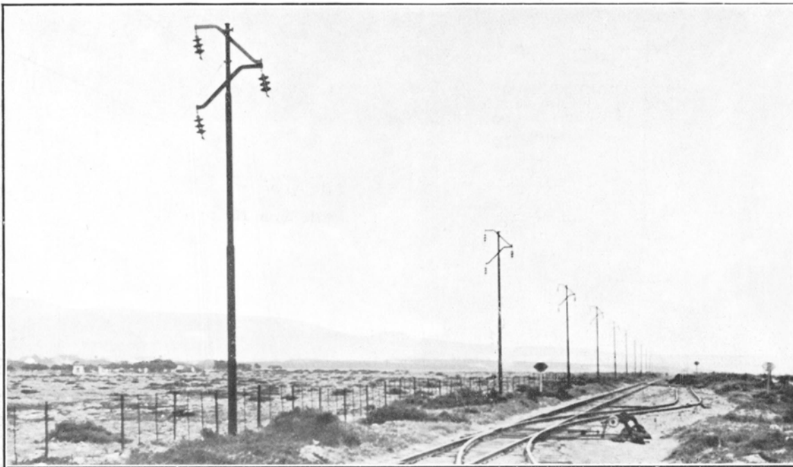
33 K.V. Transmission Line. Capetown Undertaking.
