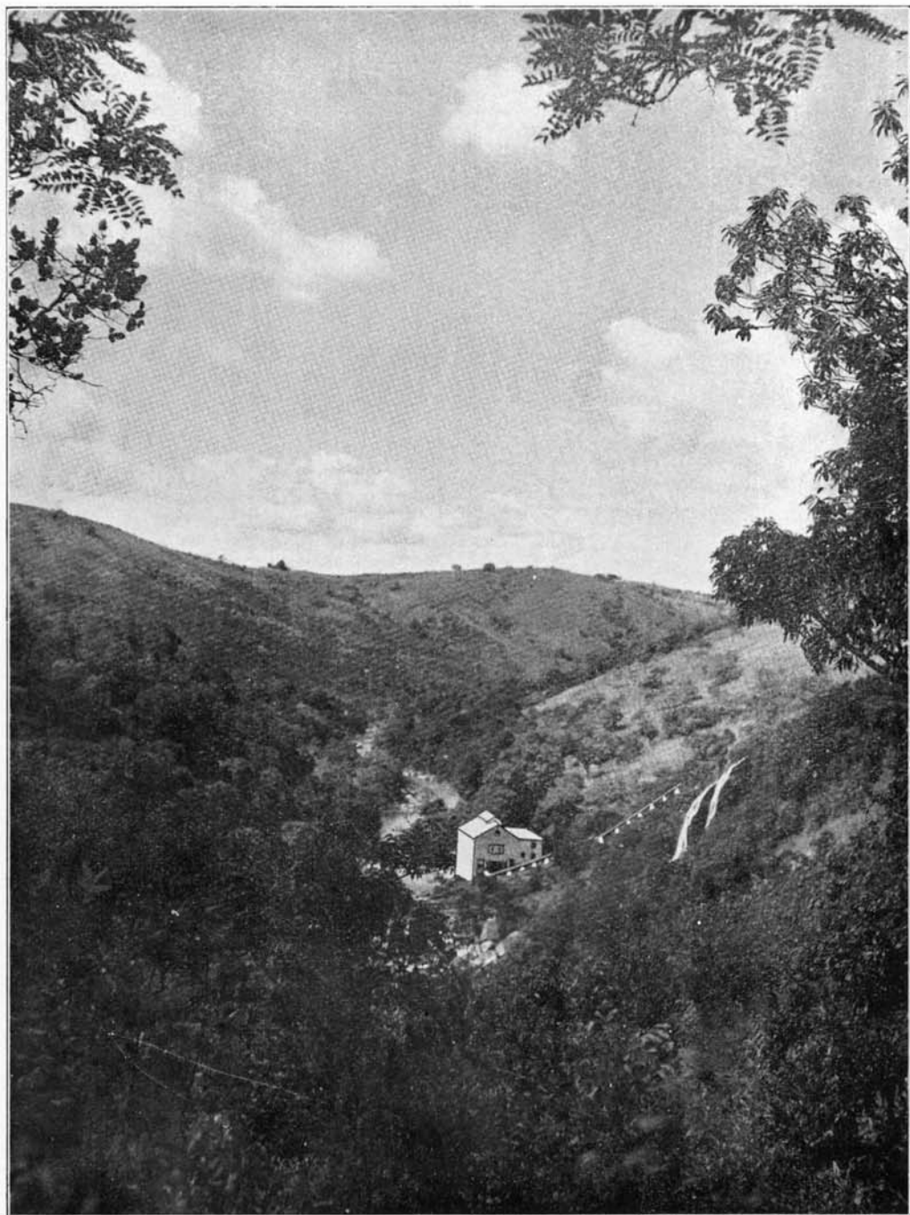
Sabie Gorge Hydro-Electric Power Station, Eastern Transvaal.
