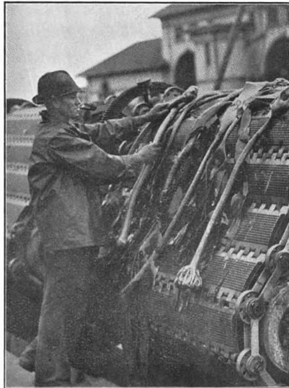
Bottom Right: Portion of Seaweed removed from the Intake Pits and Screens.
