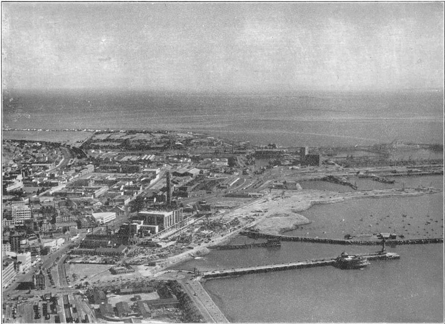
Aerial View of Table Bay Power Station showing its relation to Foreshore.
