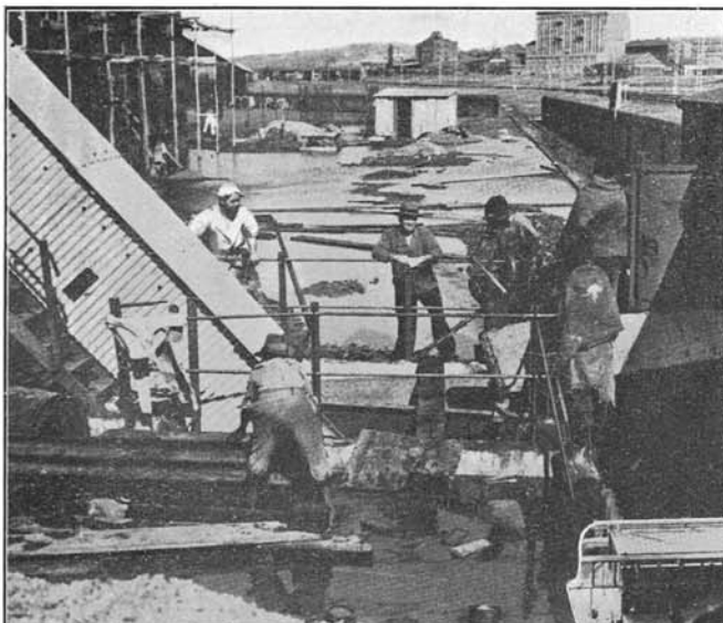
Flooding at Congella Power Station, 3rd August, 1937.
