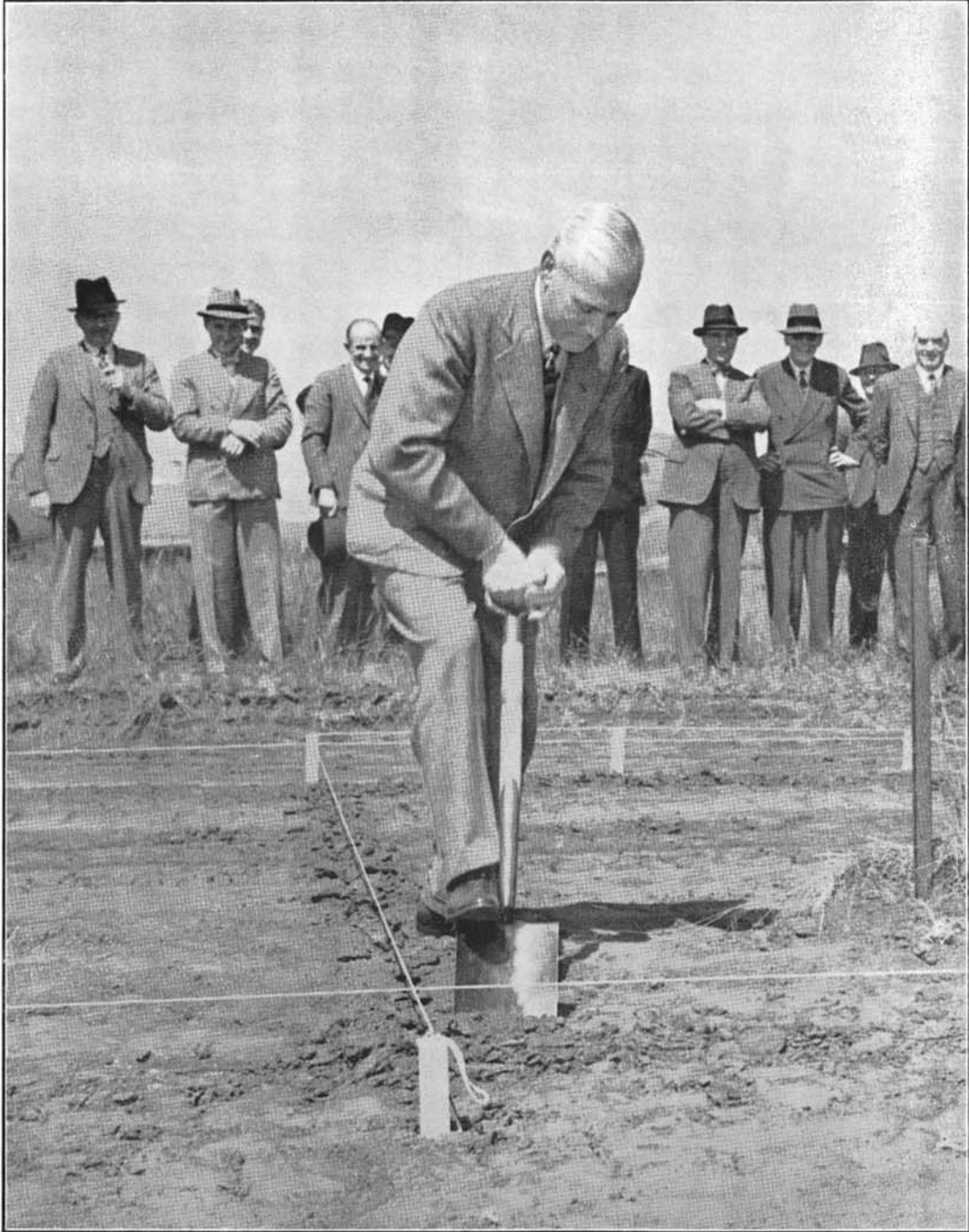
Dr. H. J. van der Bijl inaugurating construction of the Vaal Power Station, March, 1939.
