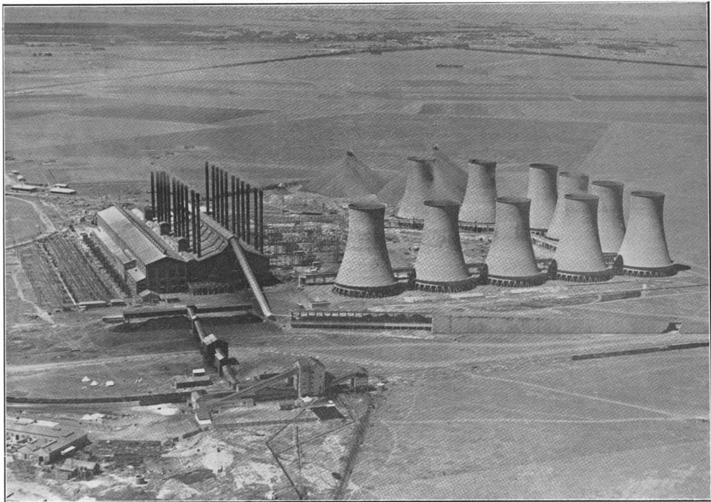
Klip Power Station showing the completed cooling system—ten hyperbolic-type cooling towers.
