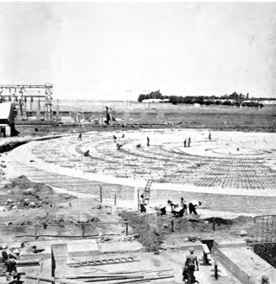
VAAL POWER STATION:
