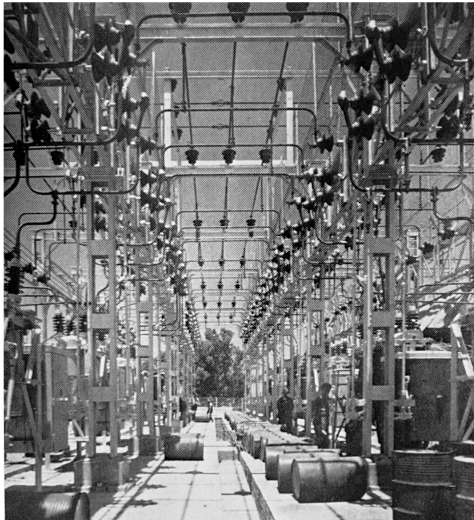
CAPE WESTERN UNDERTAKING: Oakdale substation structure under construction.
