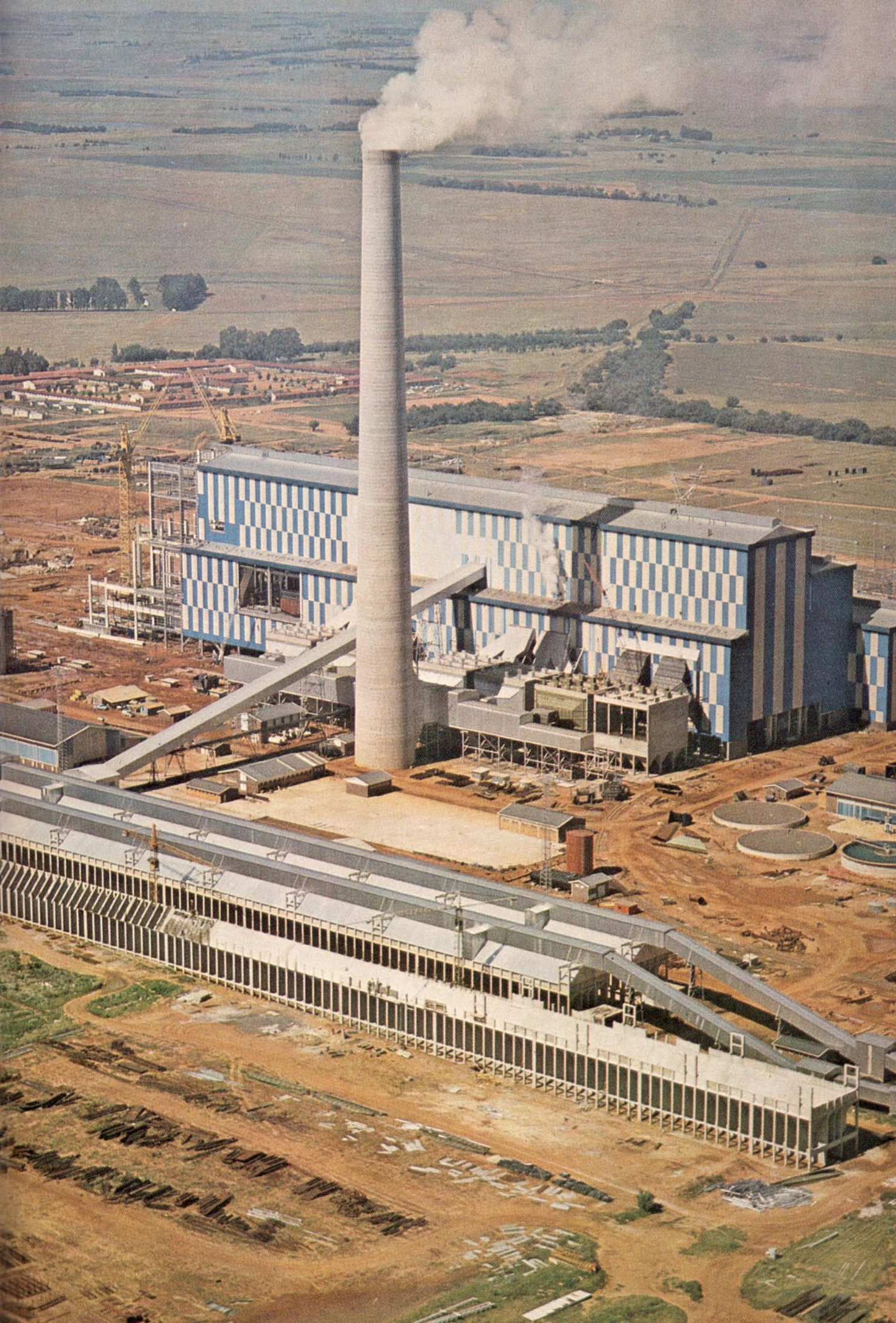
The Arnot power station in the Eastern Transvaal is the first Escom power station to operate on the reheat cycle. When complete the station will consist of six 350 MW units. The first unit reached full load in June and the second in October 1971.
