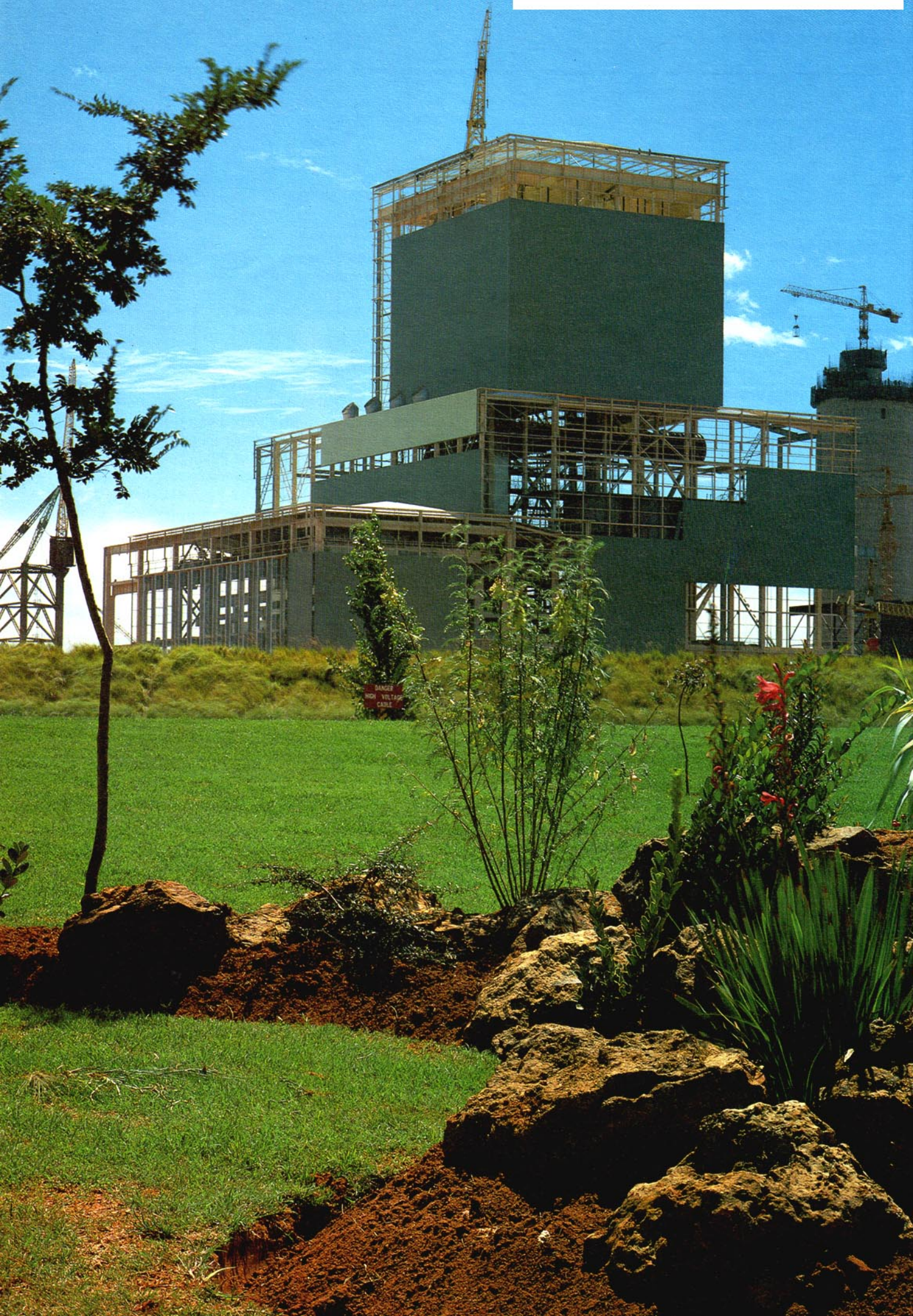
Boiler and turbine houses under construction at Duvha power station
