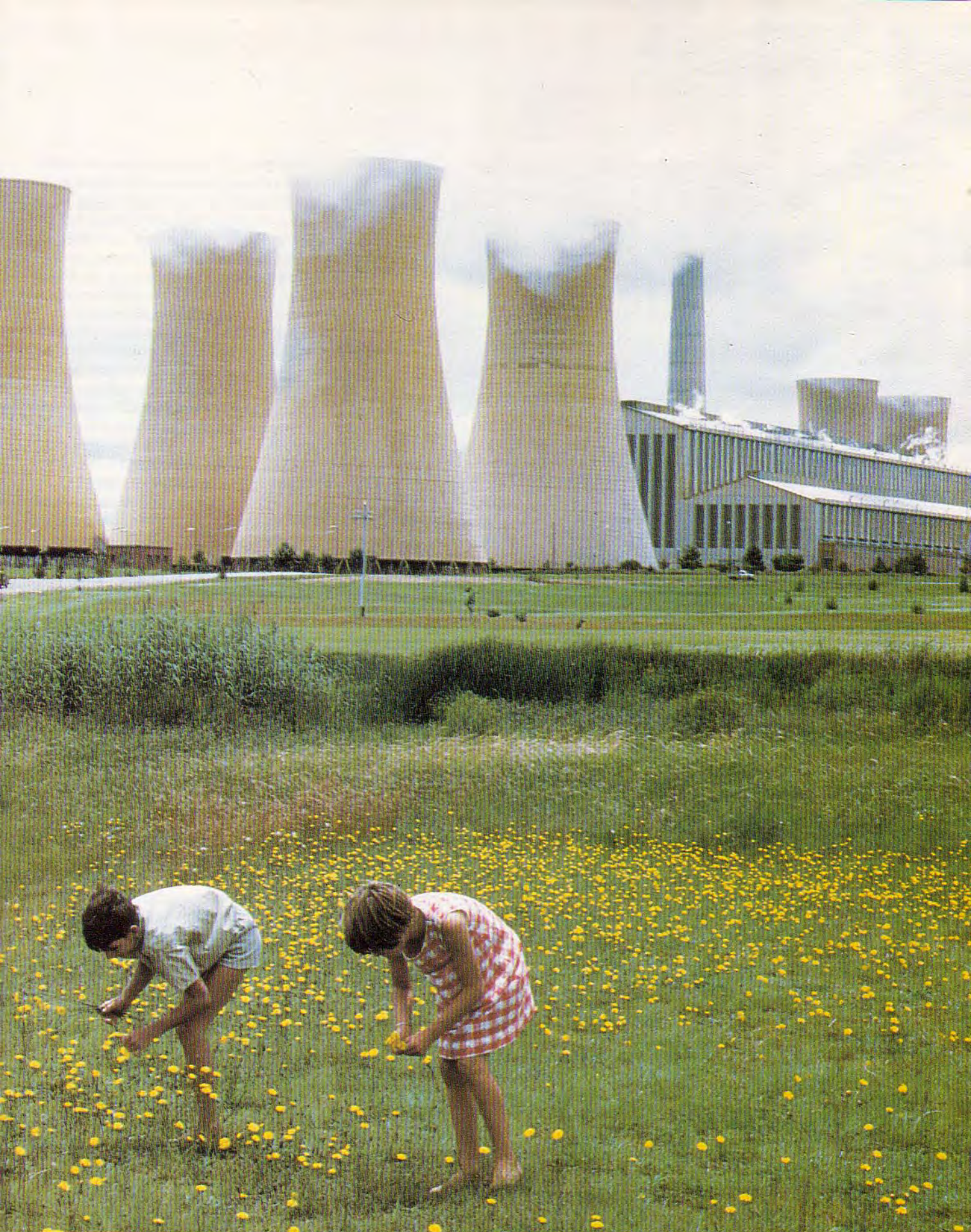
Komati, a 1 000 MW coal-fired station completed in the 1960s. Under inflationary conditions, the cost of replacing such a power station at the end of its useful lifetime of approximately thirty years can be more than 16 times its original cost. Recovery of only the historical cost of such fixed assets does not make adequate provision for financing their replacement.
