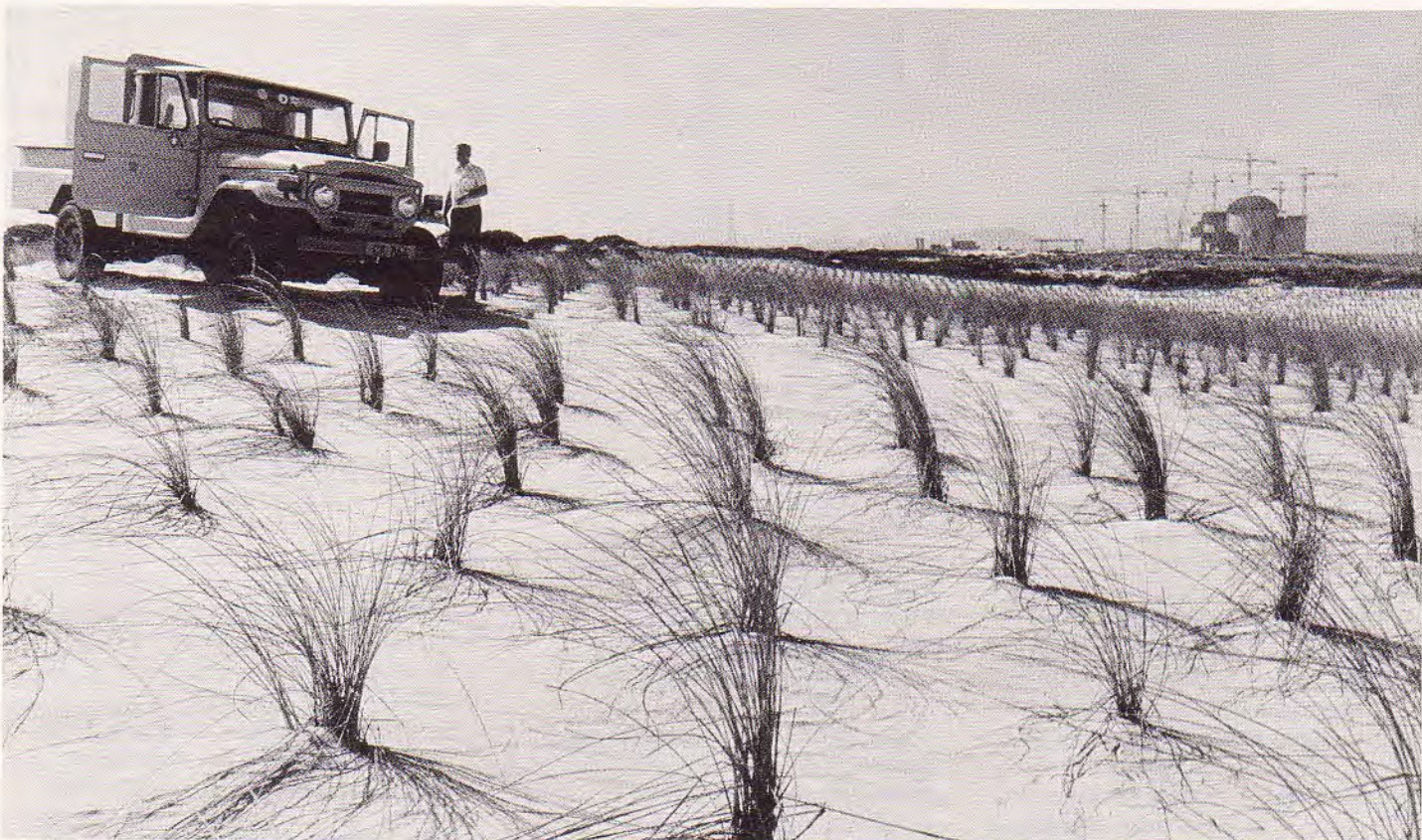
At Koeberg, Escom is involved in a project to reclaim dune wasteland. The aim is to prevent dunes from moving farther inland so destroying farmland. Similar projects are being undertaken by other organisations further up the coast.
