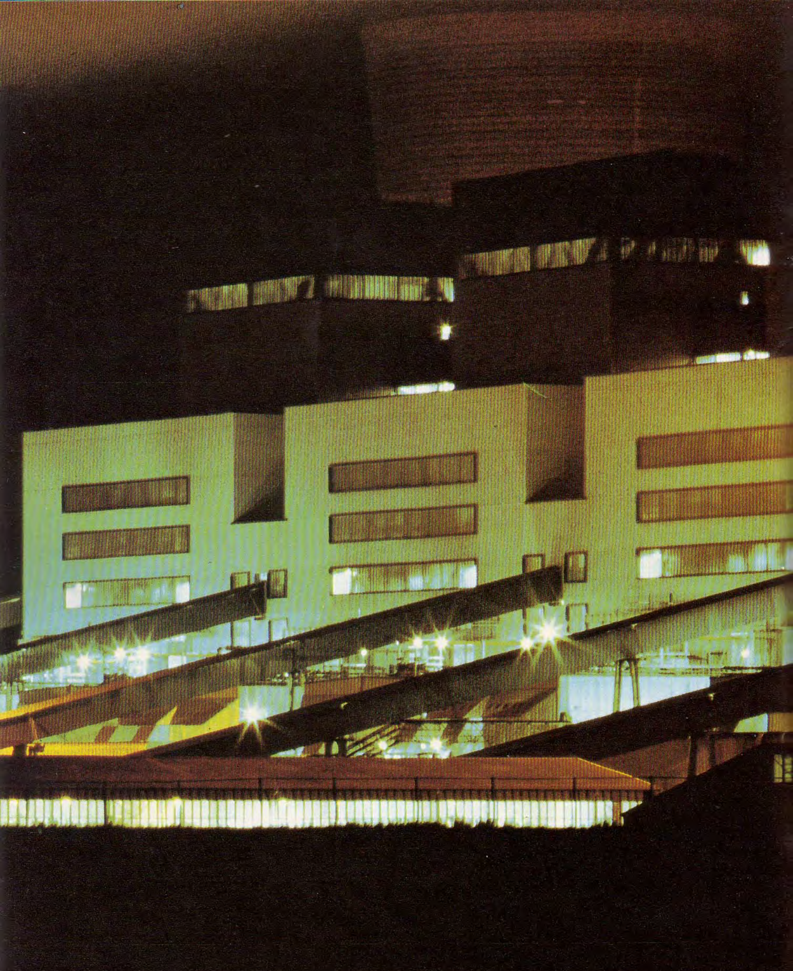
Kriel, believed to be the third largest coal-fired power station in the world, became fully operational in 1979. Planning for this 3 000 MW station began in the late 1960s and construction started in 1970. Because of the long lead times before a big, modern station is fully operational – nearly 14 years in the case of Kriel – Escom maintains development even during troughs in the business cycle.
