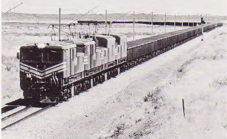
The Sishen/Saldanha electric traction system came into full operation last year; increased electrification of railways is saving the country millions of litres of diesel fuel. The substitution of electricity for oil is also taking place in diverse industrial and other applications.
