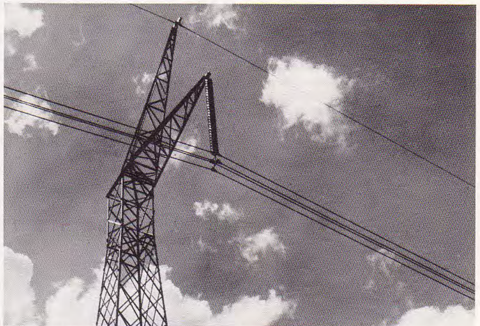
The third and final stage of the Cahora Bassa scheme became operational in 1979. A firm capacity of 1 384 MW is now available from this power station, which provided more than 10 000 million kW.h of energy to Escom during the year. Electricity is transmitted by way of 533 kV lines from Mocambique to South Africa.
