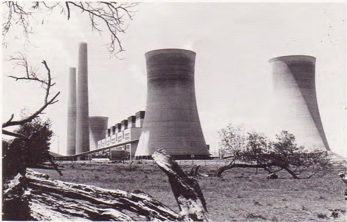
The 3 000 MW Kriel power station, which became fully operational in November, set an all-time record with a production of some 15 200 million kW.h for the year. Coal-fired stations produced nearly 87 per cent of the electricity required for the Escom system in 1979, burning more than 43 million tons of coal.
