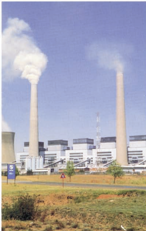
Right: Flue-gas conditioning in the stack on the right hand ensures a visible reduction in particulate emissions.
