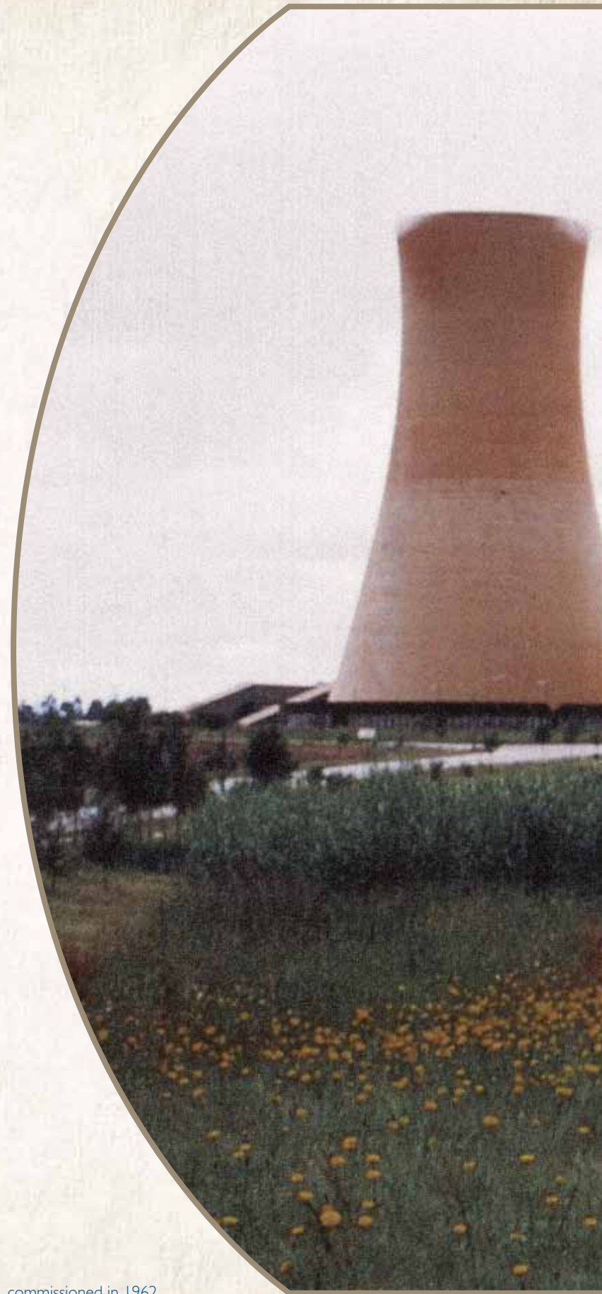
Komati Power Station, commissioned in 1962
