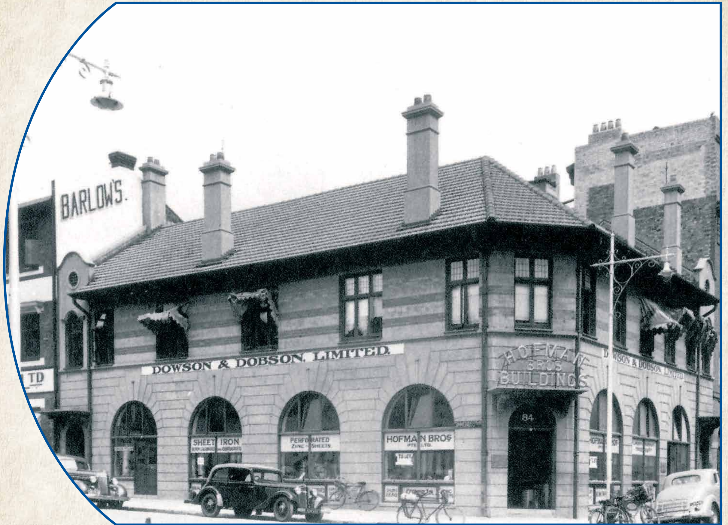
ESCOM's first headquarters, Hofman's Building, Johannesburg
