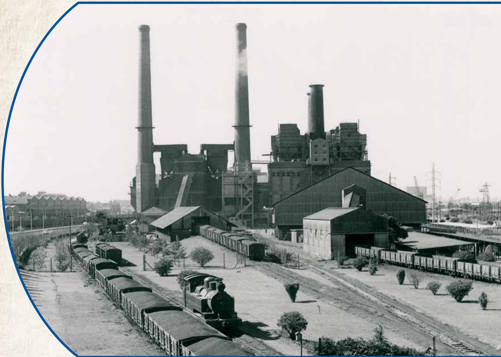
Congella Power Station
