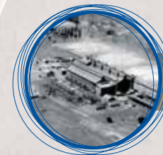
Witbank Power Station 1926
