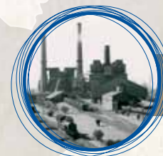
Congella Power Station 1928
