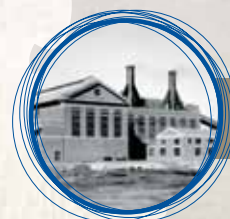
Salt River Power Station 1928
