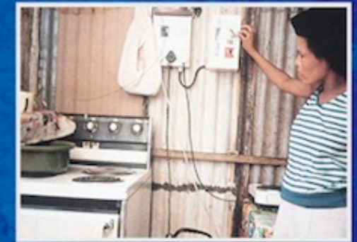
Readyboards made it possible to have electricity in homes in informal settlements.
