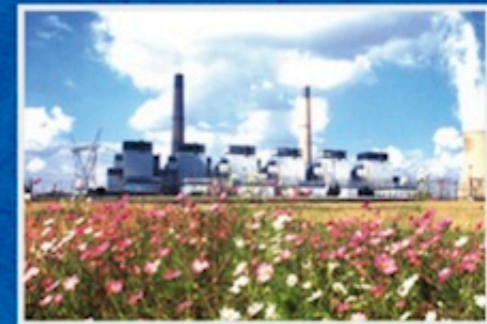
Kriel power station.
