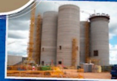
Medupi Power Station under construction.
