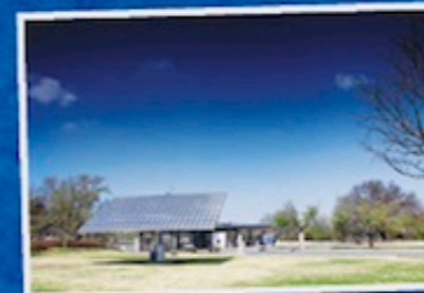
Photovoltaic panels on the Megawatt Park premises.
