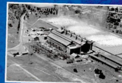
Witbank Power Station
