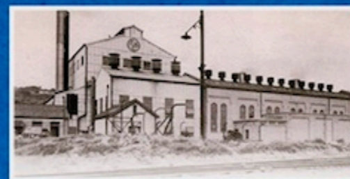
West Bank Power Station.
