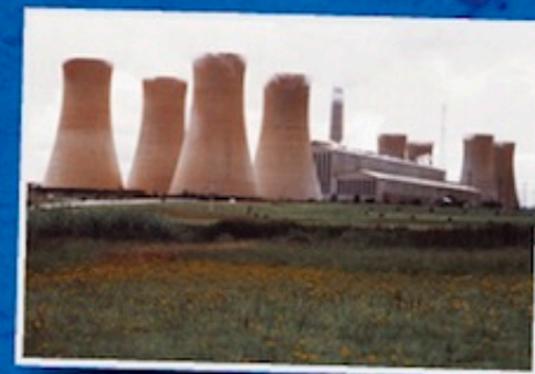
Komati Power Station.
