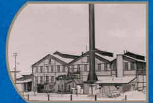
King William's Town Power Station.
