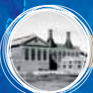
Salt River Power Station 1928
