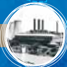
Colenso Power Station 1926
