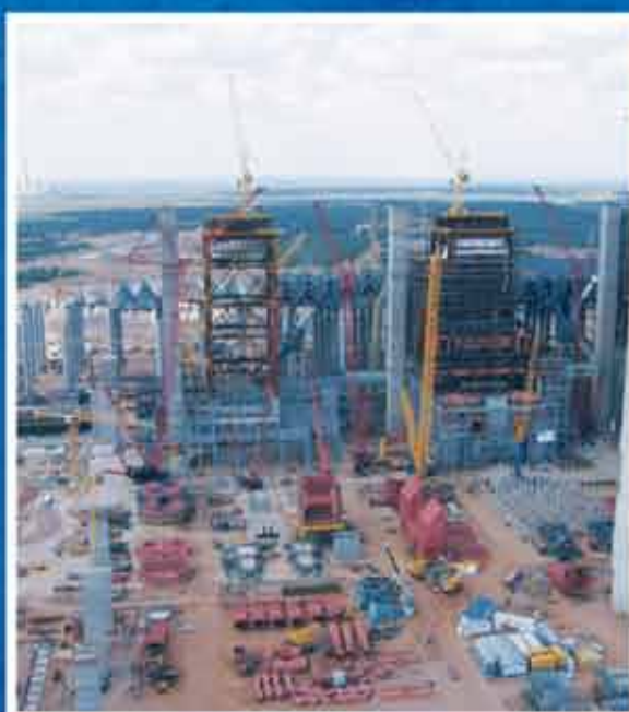
Medupi Power Station under construction.
