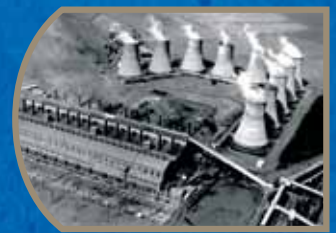
Construction of Klip Power Station began in 1934.
