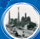
Congella Power Station 1928
