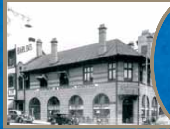
ESCOM's first headquarters, Hofman's Building, Johannesburg.
