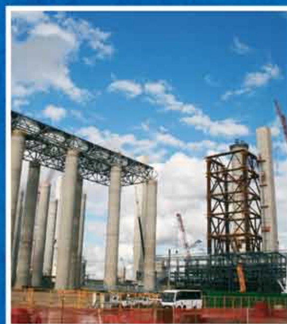
Kusile Power Station under construction.
