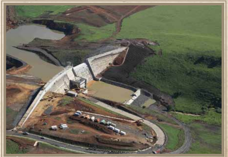
Braamhoek Dam - Ingula Pump Station
