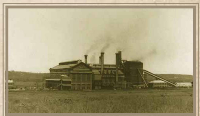
Congella I Power Station before World War 2
