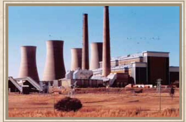
Ingagane Power Station
