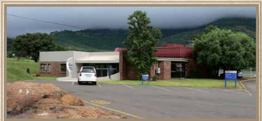
Drakensberg Pump Station
