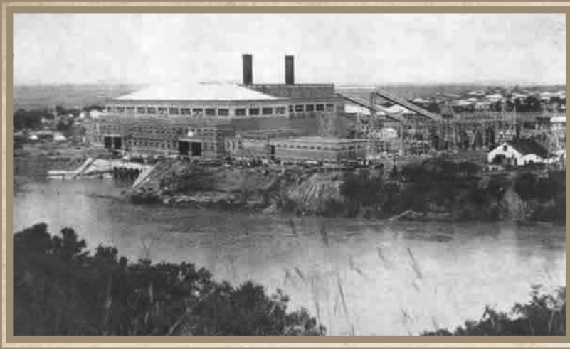
View showing the original cooling water intake works set back from the river bank. This silted up while the station was still being commissioned and a new intake was constructed.
