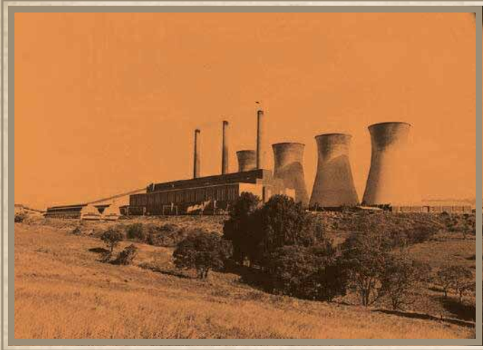
Umgeni Power Station
