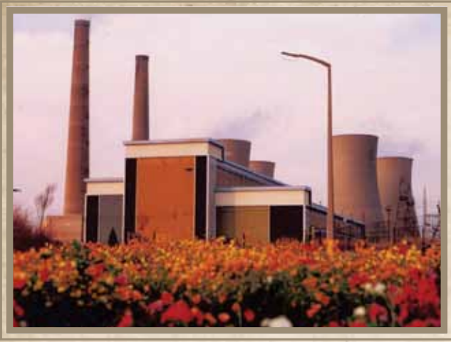
Ingagane Power Station
