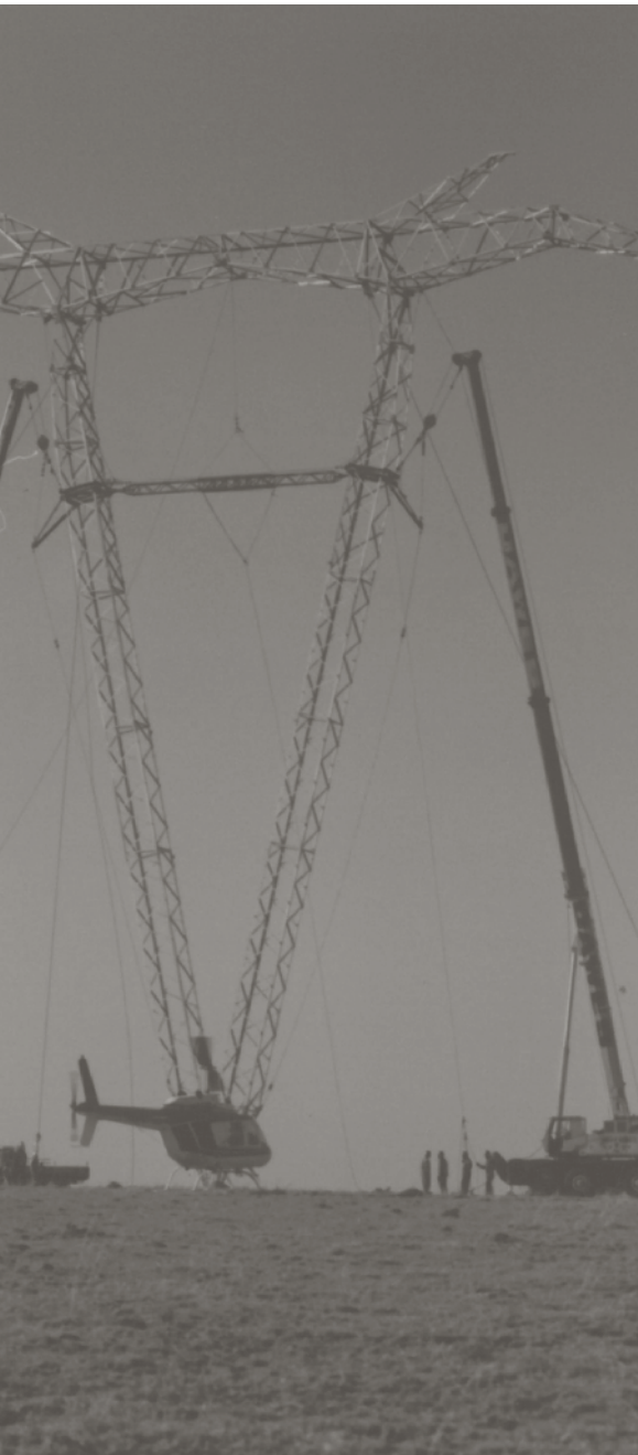
First electrification project in Lephalale
