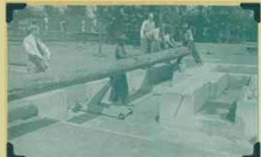
Dropping the pole into the hole
