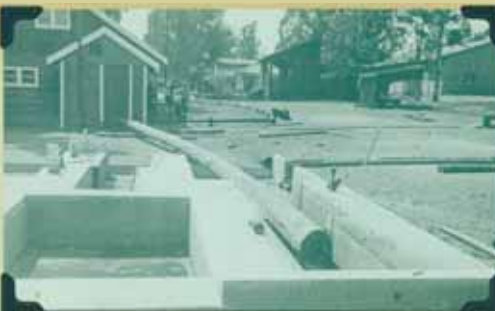
Start applying concrete
