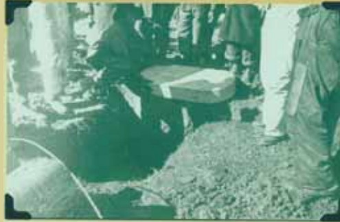
Preparing the concrete base for the pole
