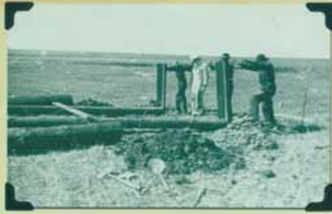
Preparing the A frame back plates
