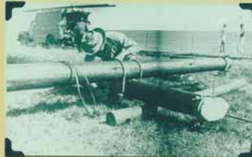
Tightening the A frame nuts
