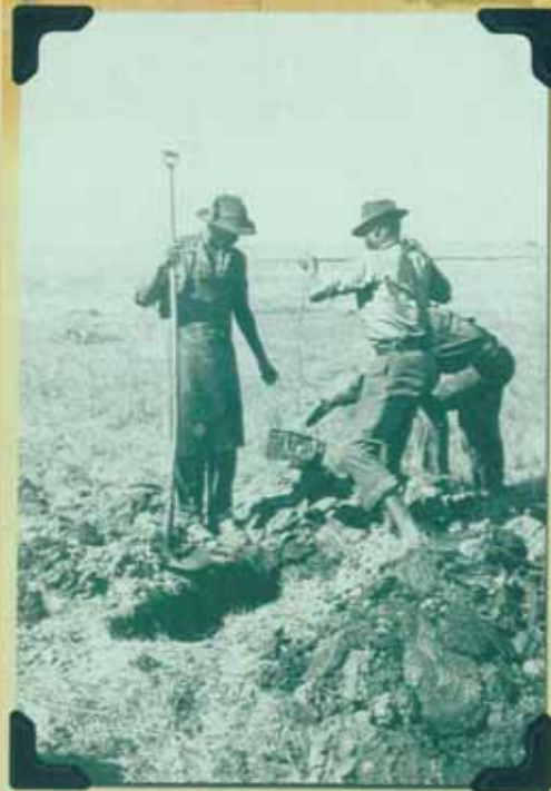
Attending to caved-in hole in vic area
