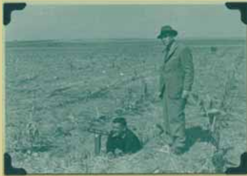
Checking that the X-arm is level
