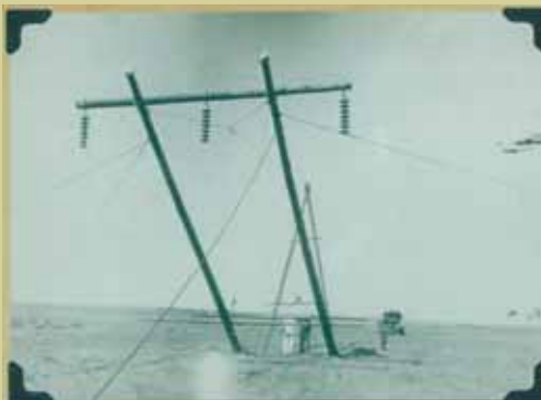
Pulling the pole with the A frame
