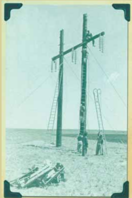
Hooking the insulators
