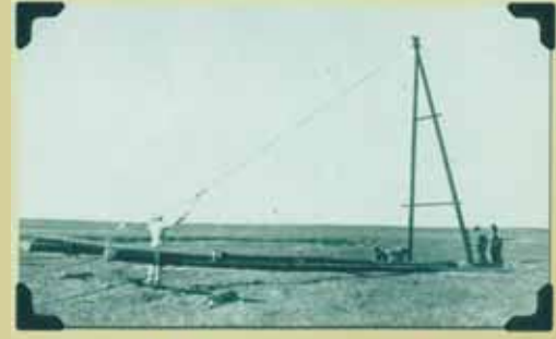
A frame in place
