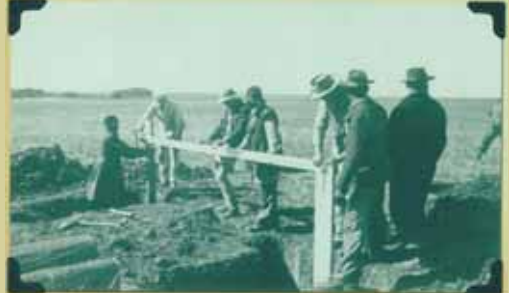
Checking that hole is level
