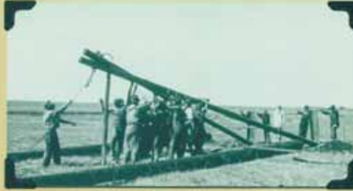
Start lifting the A frame
