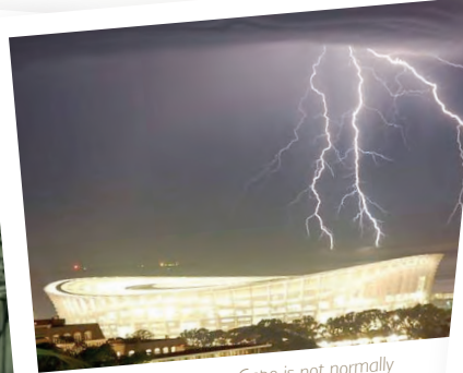
Although the Western Cape is not normally associated with thunderstorms, they do occur and can also wreak havoc as far as "dips" and "trips" are concerned.
