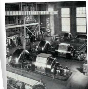
Inside the turbine house at Salt River 1 showing sets 1 to 3. These were the first steam-driven sets ordered and commissioned by Eskom.
