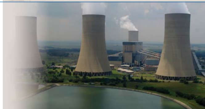
Lethabo power station in Vereeniging.
