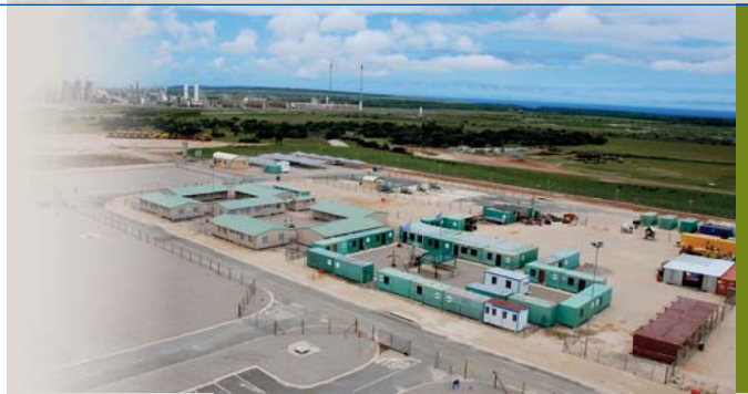
Additional units are being built at Gourikwa power station.
