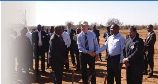
The sod turning for the new Medupi power station in Lephalale on 14 August 2007.
