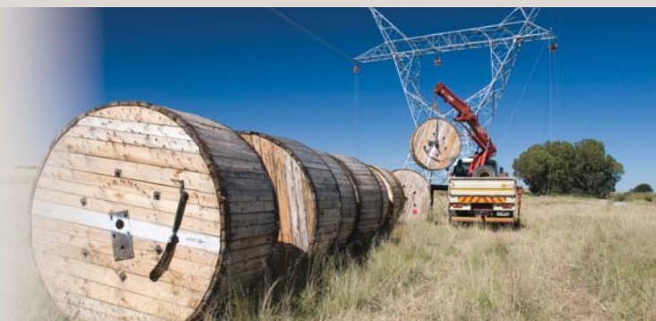
A new high-voltage transmission line being built near Bothaville.
