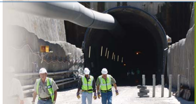
The tunnel at the new Ingula pumped storage scheme near Ladysmith.
