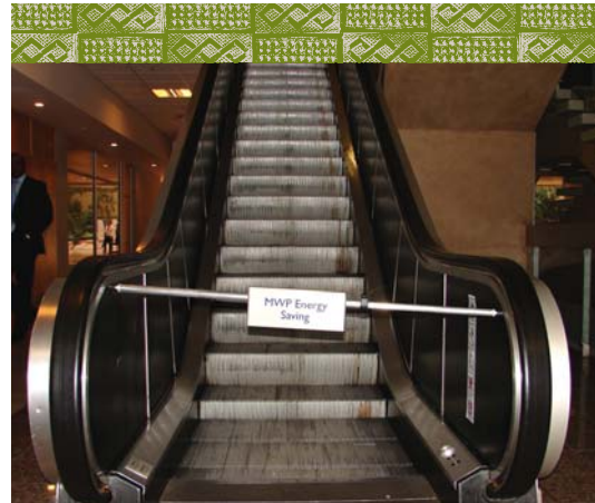
All the head office escalators were switched off to conserve energy
