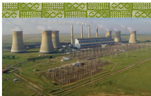
Camden power station in Ermelo is the first old coal-fired station successfully returned to service
