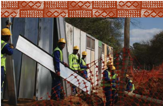
Temporary housing is built for construction workers in Lephalale
