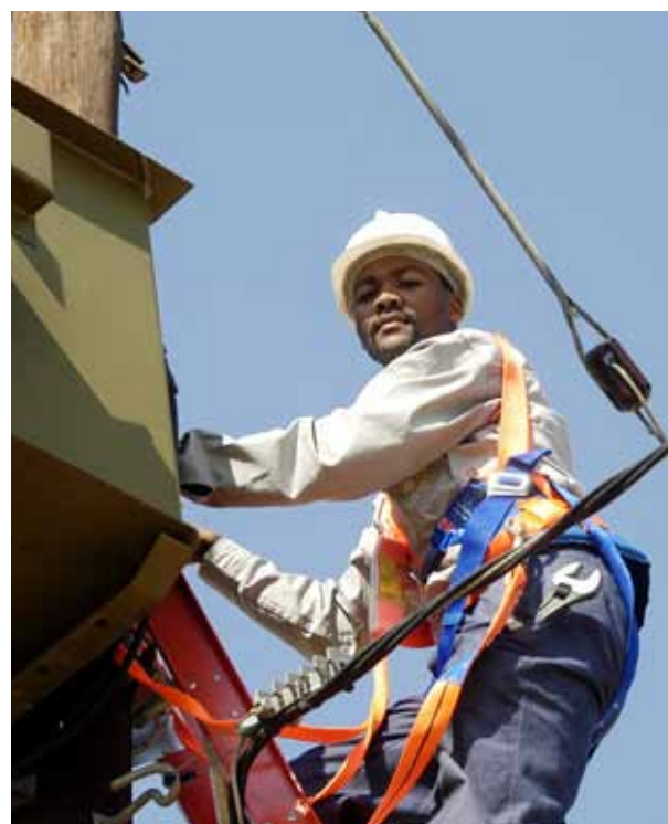
Eskom workers maintain around 390 000km of power lines across the country.
