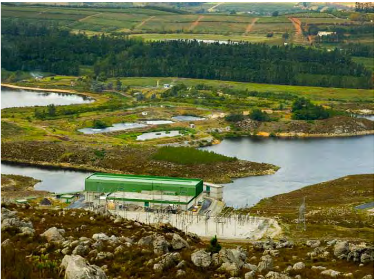
Palmiet pumped-storage scheme near Grabouw in the Western Cape.
