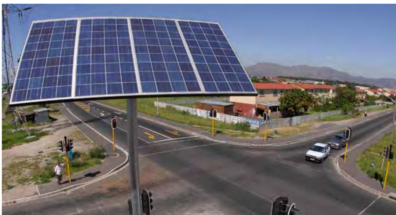
A demonstration solar-powered traffic light in the Western Cape.
