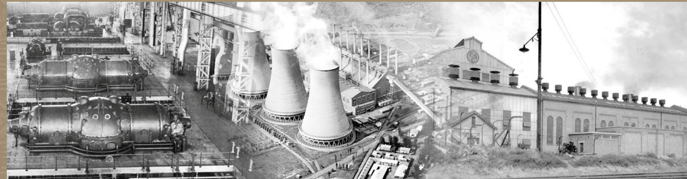
Vaal River Power Station, giant turbines
