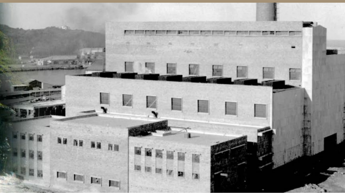
West Bank 1 Power Station
