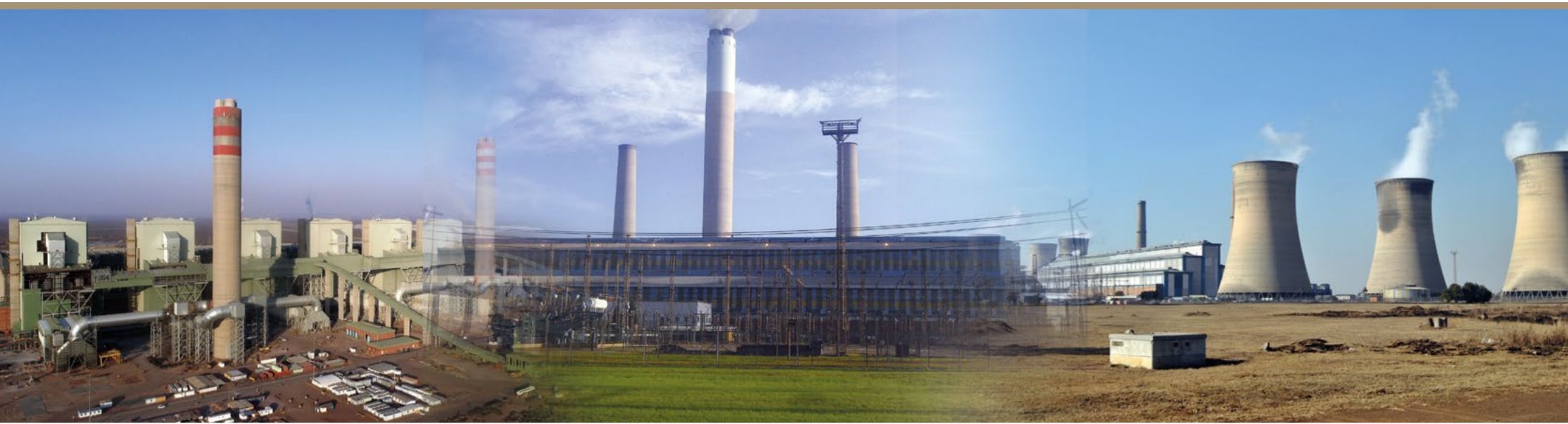
Medupi Power Station
