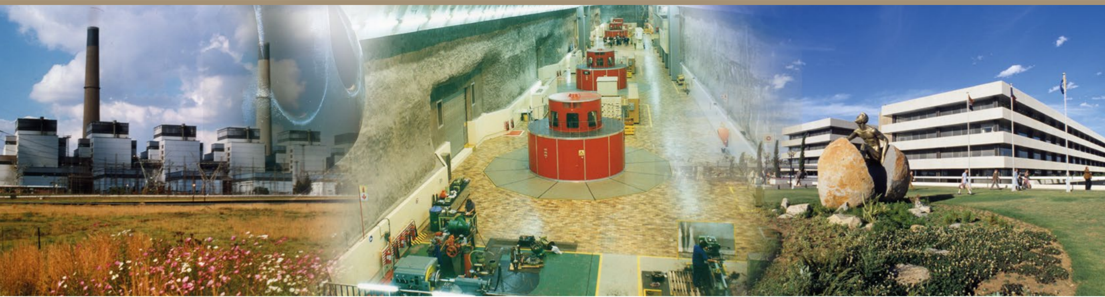
Kriel Power Station
