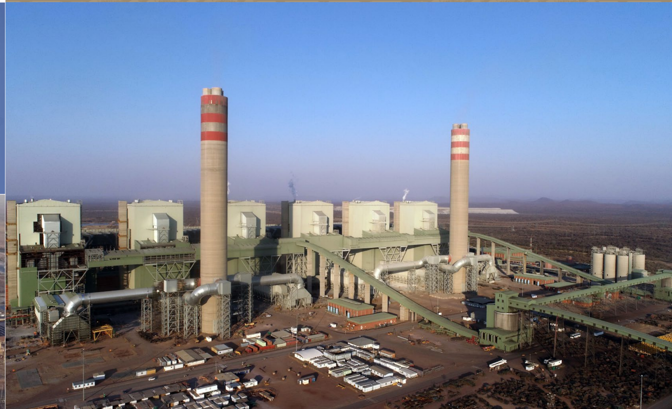
Medupi Power Station
