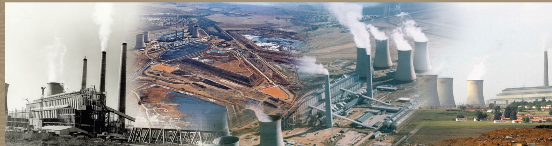
Camden Power Station
