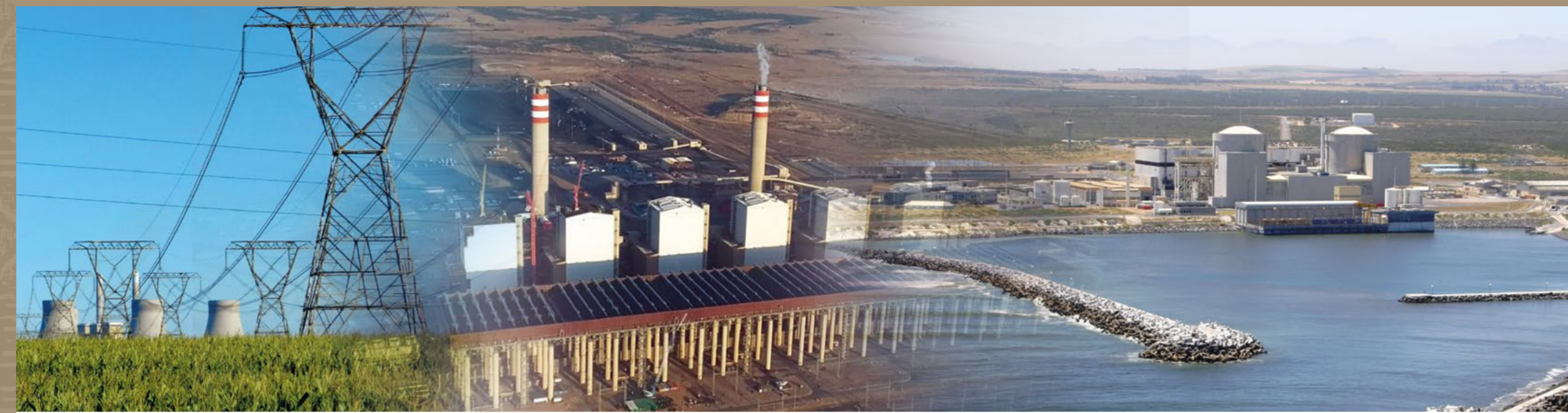
Kusile Power Station
