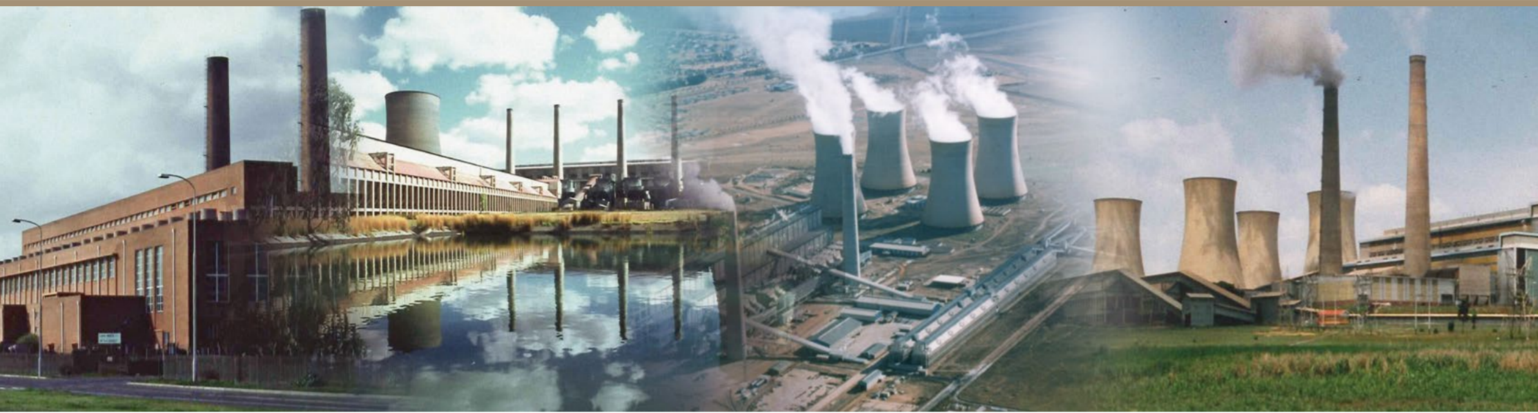
Salt River 2 Power Station
