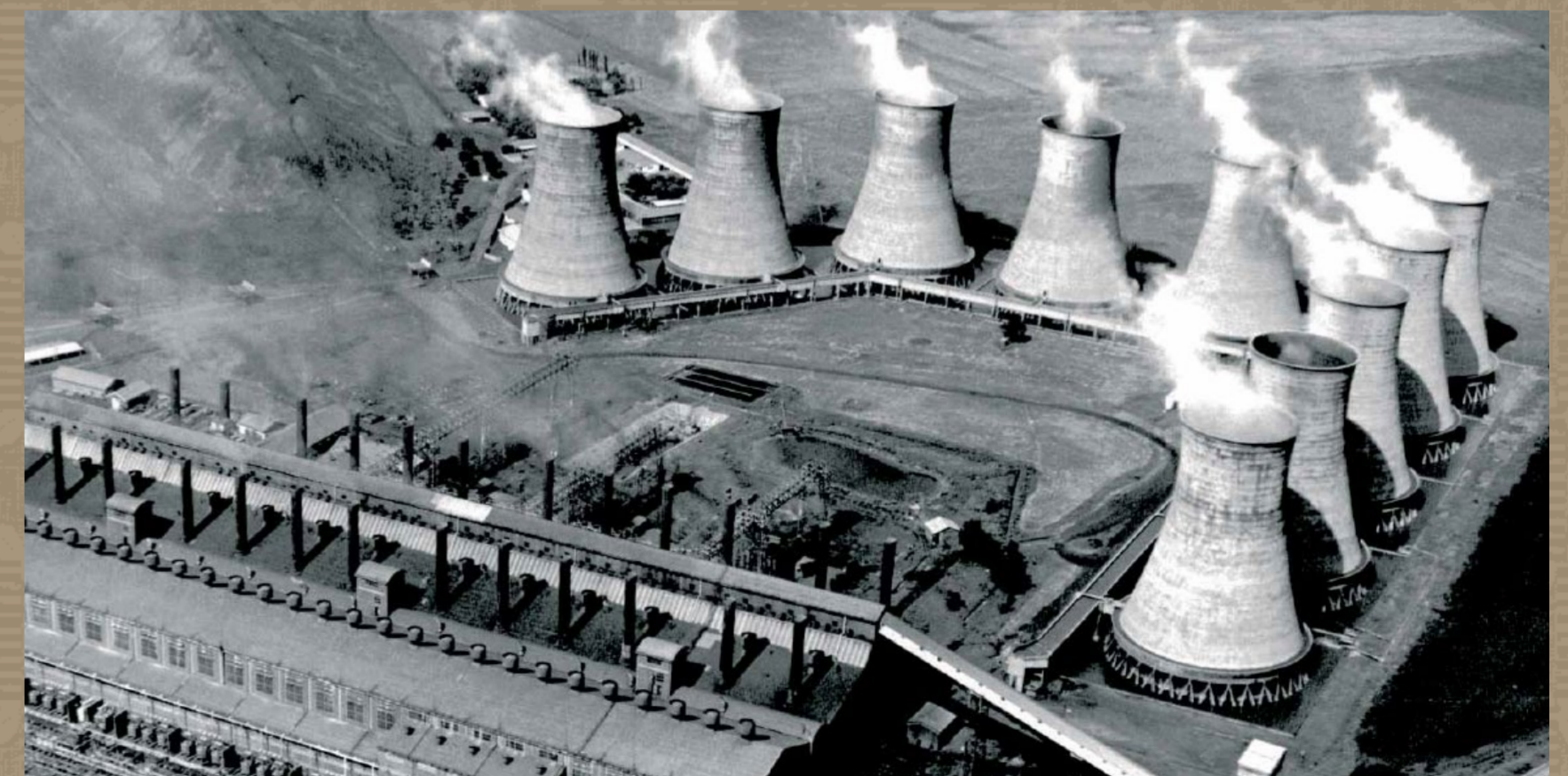
Klip Power Station after completion
