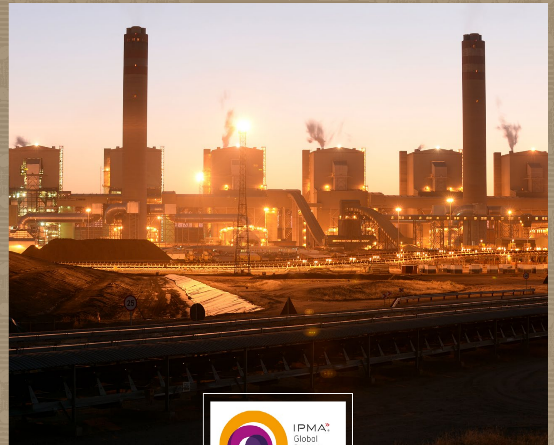
Medupi Power Station
