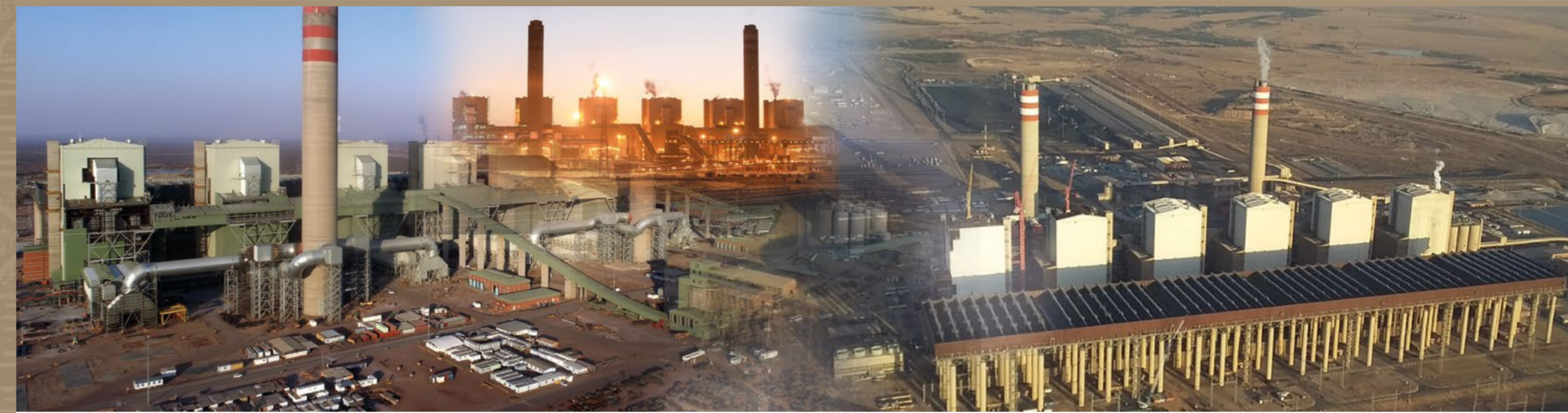
Medupi Power Station
