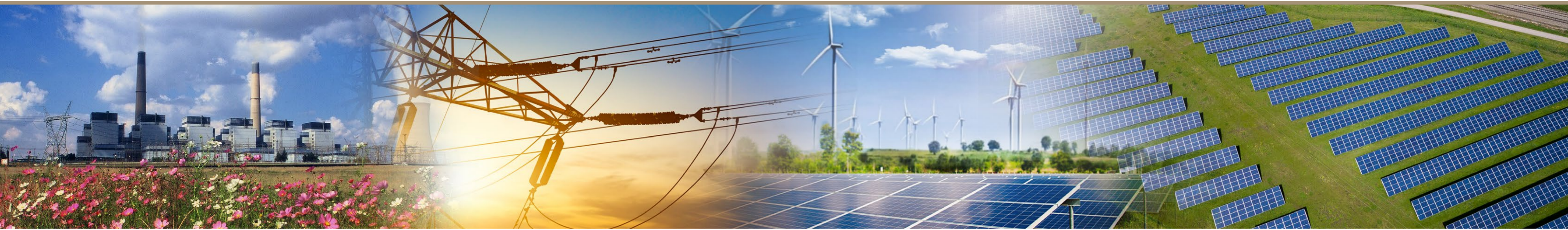
Kriel Power Station
