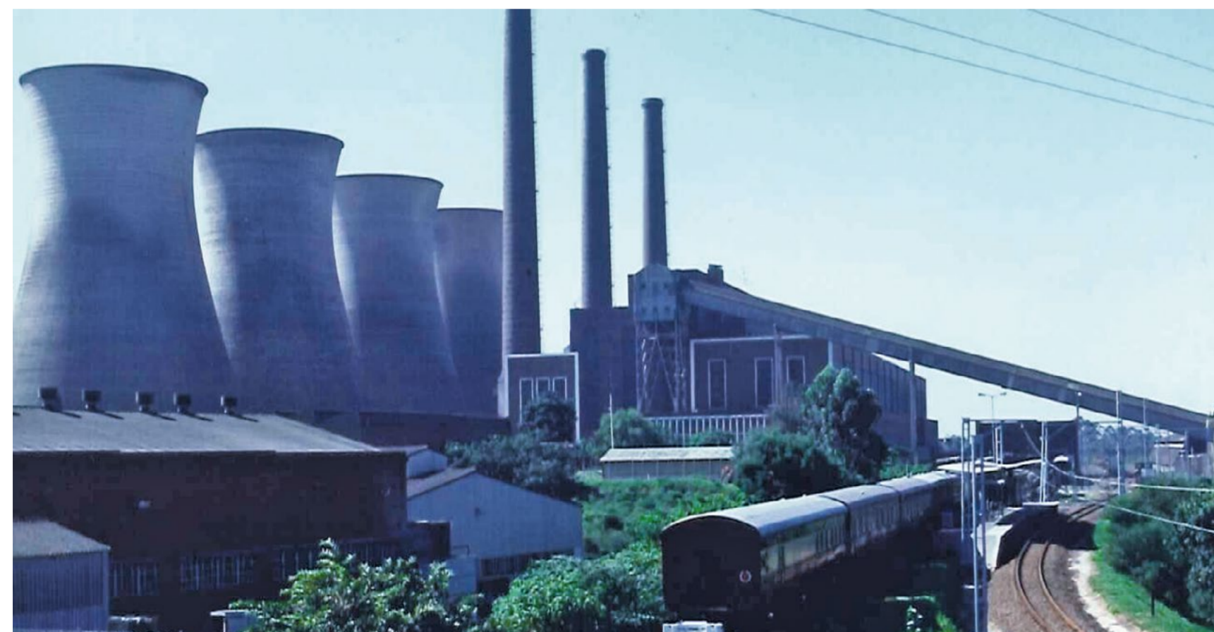
Umgeni Power Station, KwaZulu-Natal
