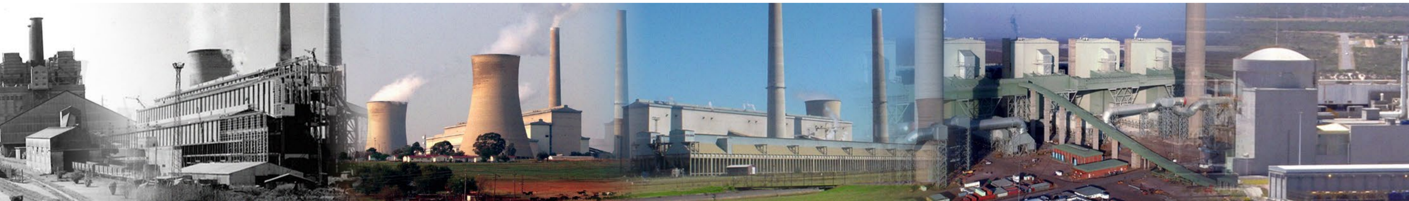
Congella Power Station
