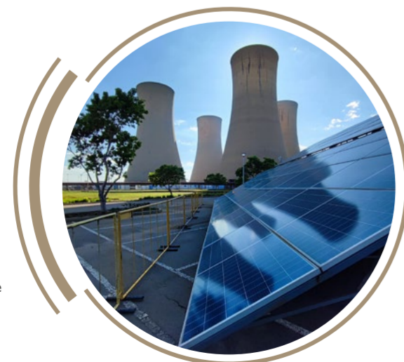
Photovoltaic panels at the Komati Power Station
