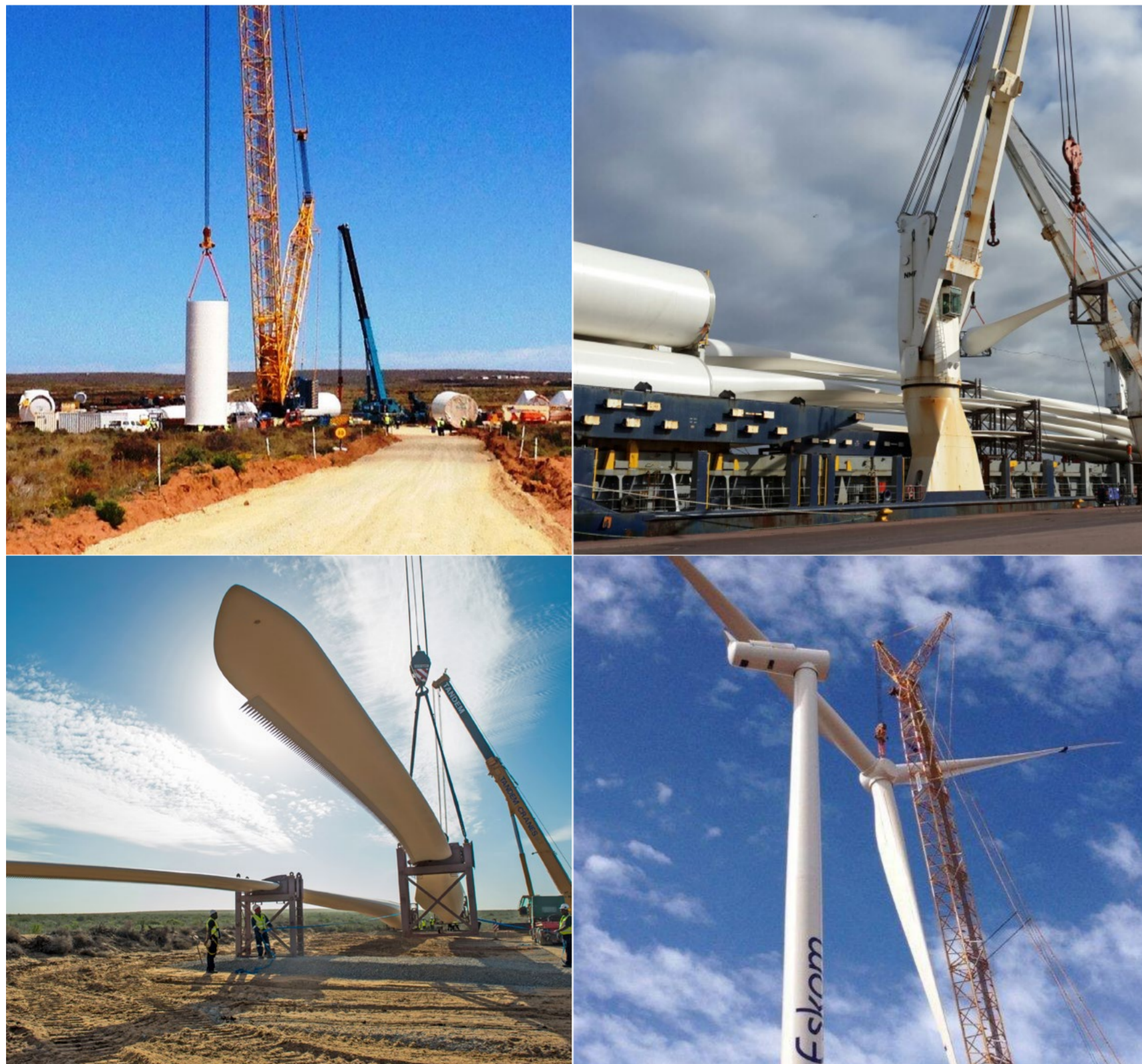
Constructing the Sere Wind Farm
