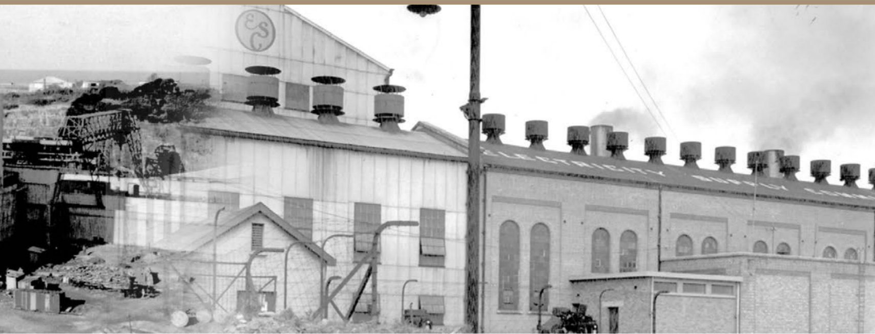
West Bank 2 Power Station, Eastern Cape Province
