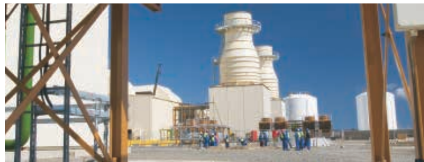
Ankerlig open cycle gas turbine station in Atlantis near Cape Town
