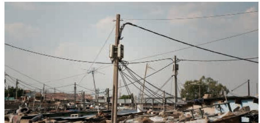
Illegal connections not only create revenue problems for Eskom, but also create safety risks
