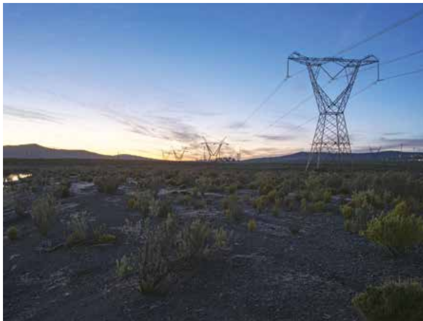
Eskom operates around 359 337km of power lines across South Africa
