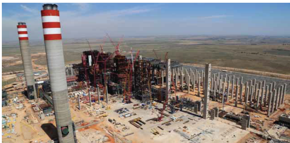
Kusile Power Station in Mpumalanga, once completed, will be one of the largest dry-cooled coal-fired power stations in the world
