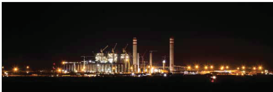
In order to accelerate progress on the Medupi Power Station Project, additional shifts were introduced, 24 hours a day, seven days week. Unit 6 reached its full load of 794MW on 26 May 2015
